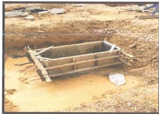
Photo 3.14: Formwork of pile cap.
