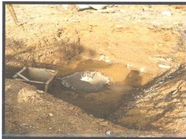
Photo 3.12: 50 mm Lean Concrete
