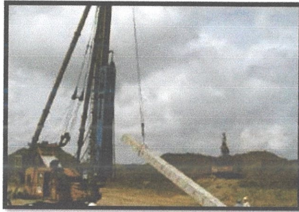
Photo 3.4: Lifting pile.
