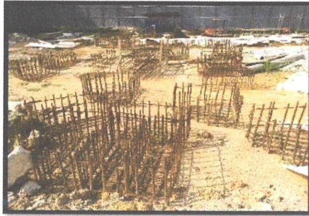
Photo 3.13: Basket of Reinforcement bar.
