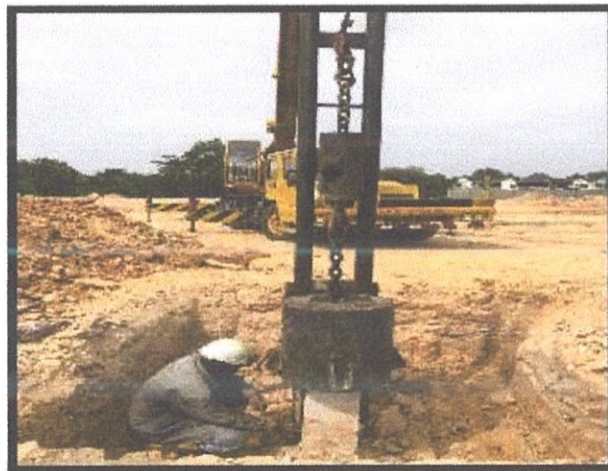
Photo 3.9: Pile Driving Analyzer (PDA).
