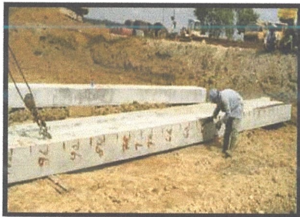
Photo 3.3: Marked pile.
