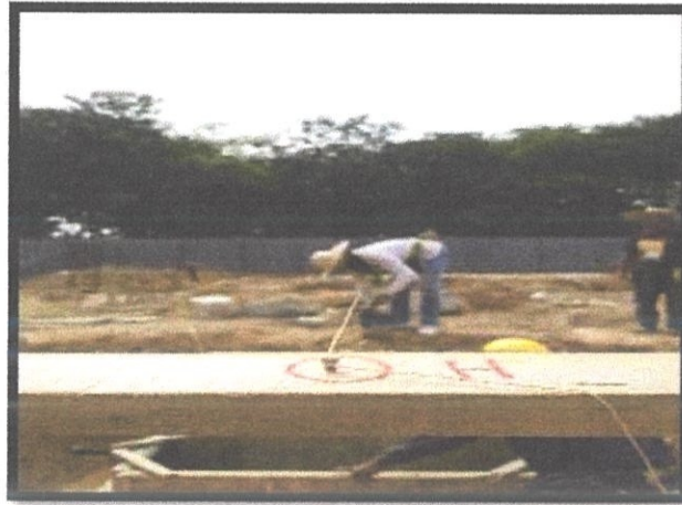
Photo 3.11: A thread for grid line.
