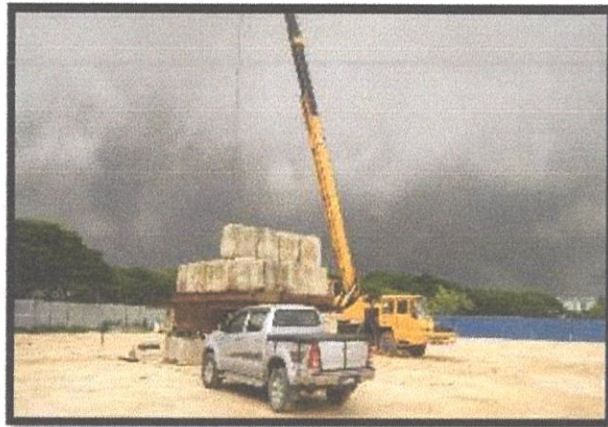
Photo 3.10: Maintained Load Test (MLT).
