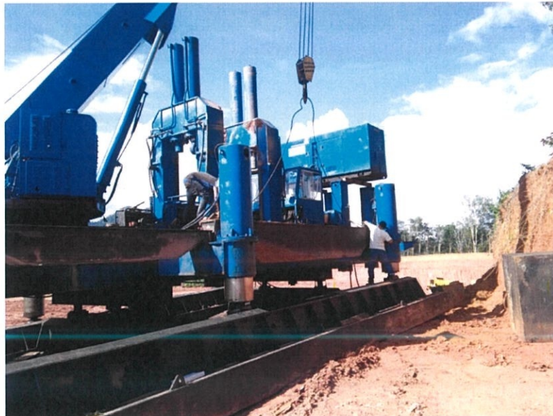
Figure 3.25 Placing counterweight beam
