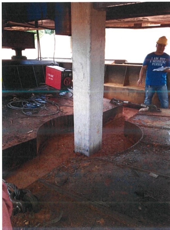
Figure 3.34 Jacked in pile
