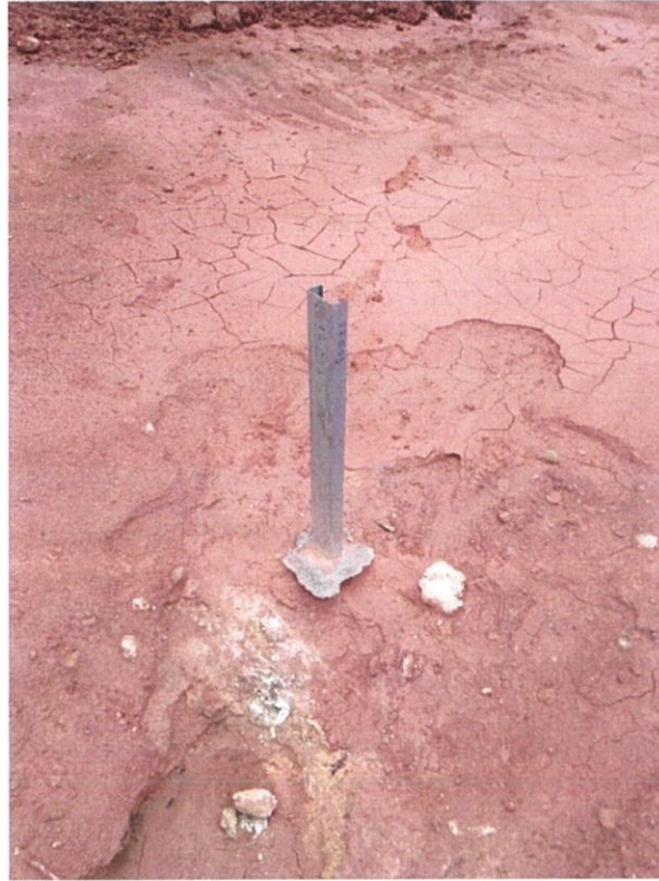
Figure 3.5 Peg level that has been marked by surveyor
