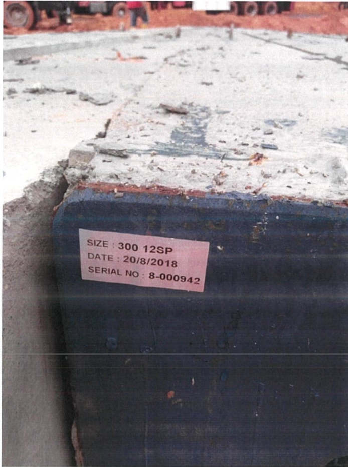
Figure 3.42 Tag on piles
