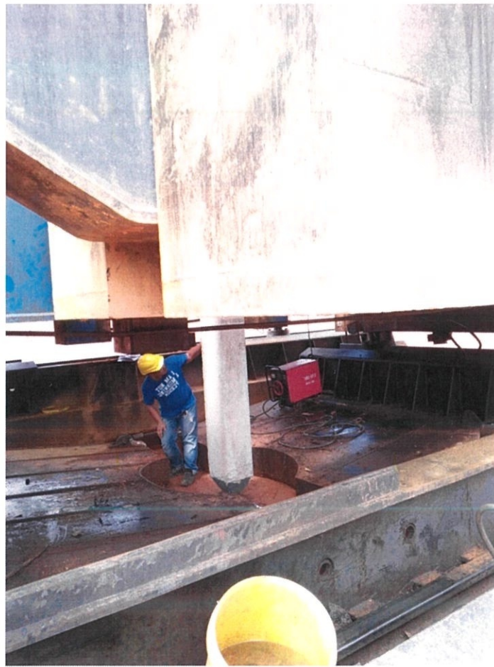
Figure 3.32 Positioning the pile to the point
