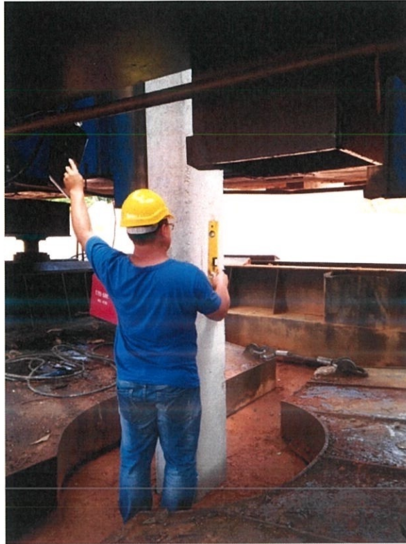
Figure 3.33 Checking pile stable using spirit level
