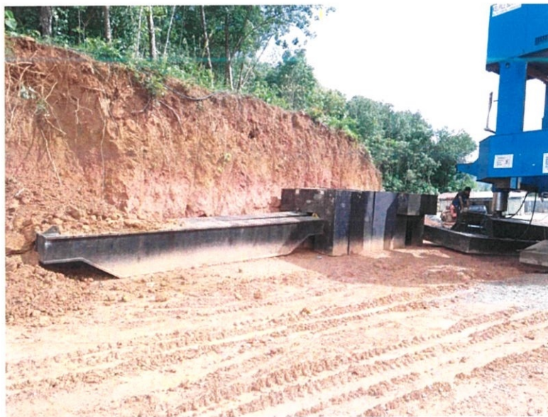
Figure 3.23 Counterweight beam and F-counterweight
