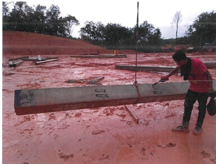
Figure 3.30 Markings the piles
