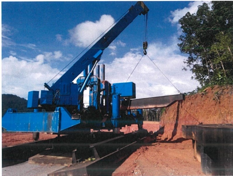
Figure 3.24 Lifting counterweight beam
