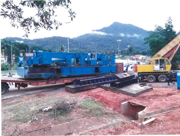
Figure 3.17 Placing main body
