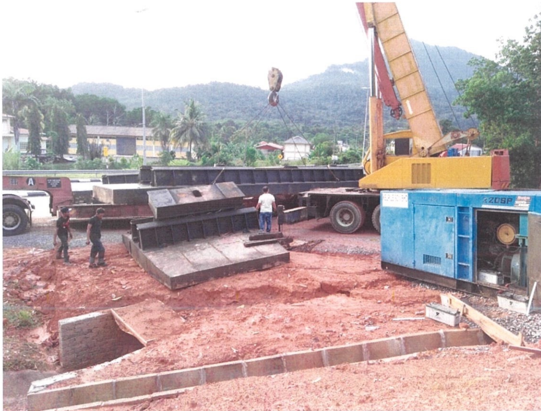
Figure 3.16 Placing long boat at ground
