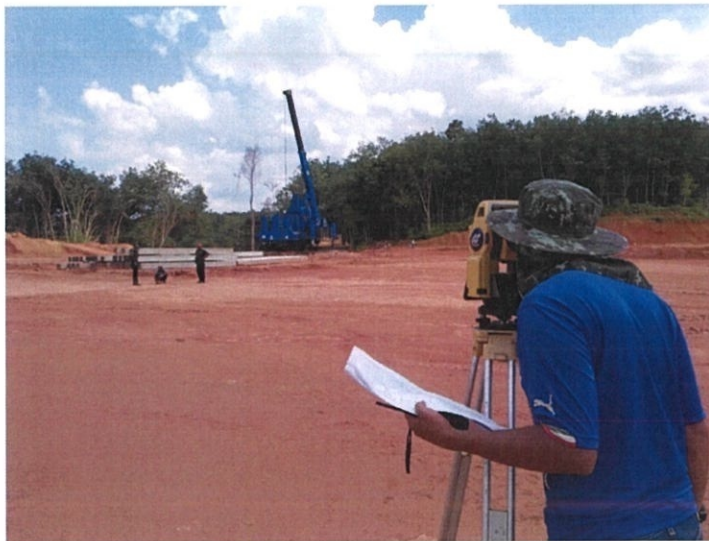
Figure 3.4 Surveyor taking read on RL level
