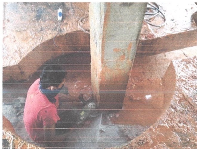
Figure 3.39 Cutting pile
