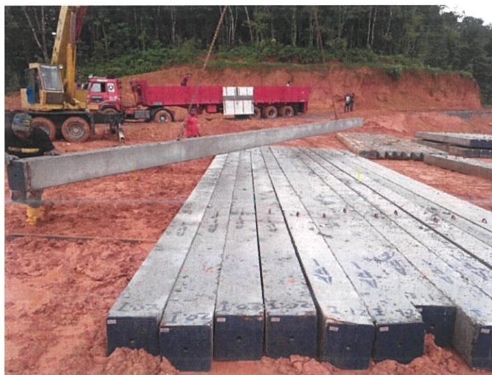
Figure 3.41 Precast pile API arrived at site
