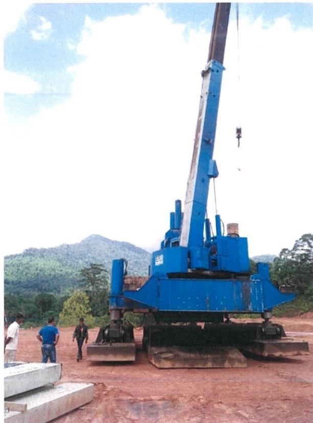
Figure 3.28 Pile machine moving to piling point
