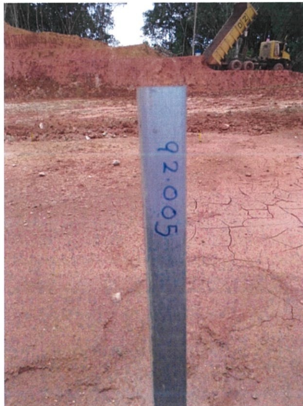
Figure 3.6 Current RL that had been marked by surveyor
