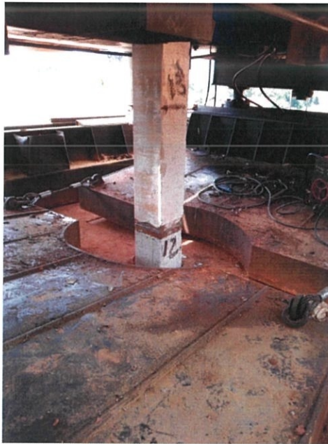
Figure 3.35 Jointed extension piles
