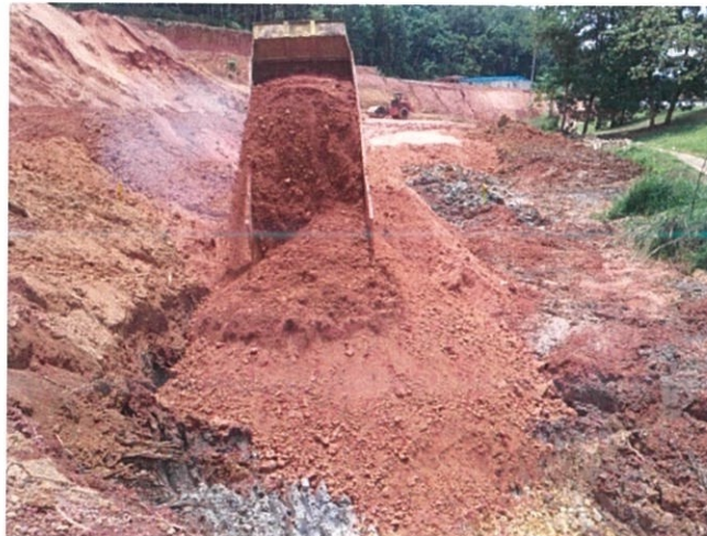
Figure 3.8 Dump soil at filling area
