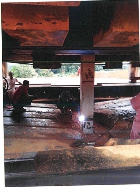
Figure 3.36 Welding extension pile
