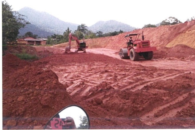
Figure 3.9 Compacting filling area
