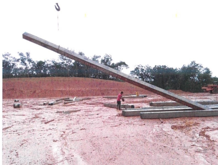
Figure 3.31 Lifting piles
