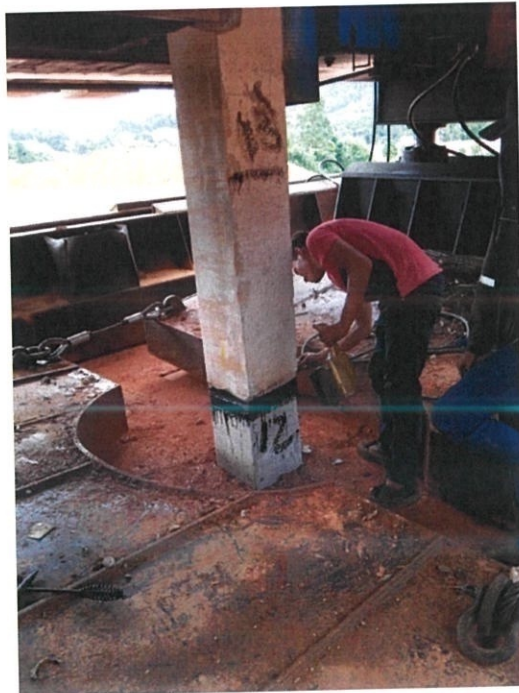
Figure 3.37 Paint bitumen on pile
