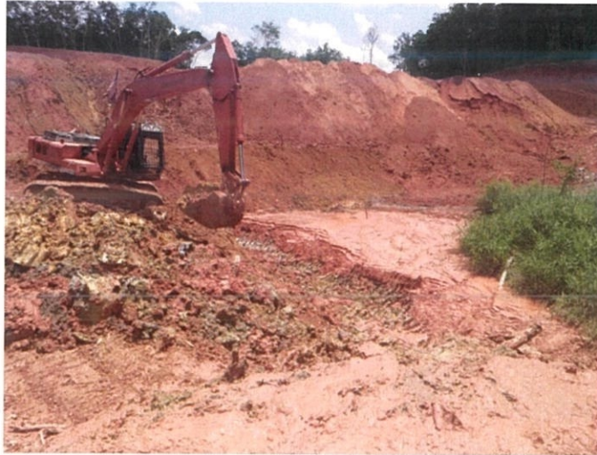
Figure 3.7 Disposal topsoil at filling area
