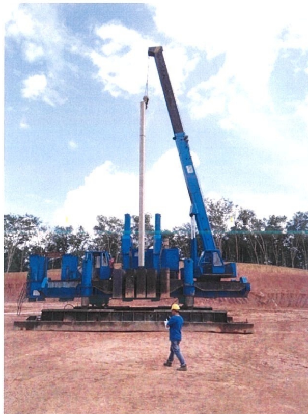
Figure 3.15 Hydraulic static pile driver
