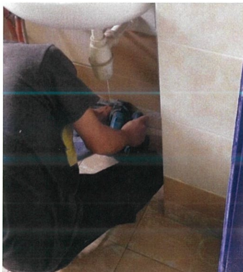
Figure 8 - Grinding process include 4 inches skirting.
