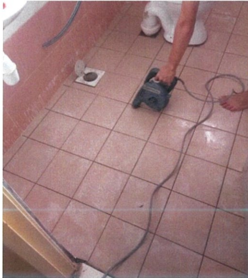
Figure 6 - Using a blower to ensure no dust left.
