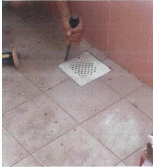
Figure 3 - Take out the trap using an iron chisel.
