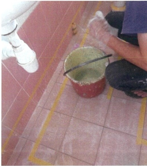
Figure 21 - The mixture are being apply on skirting.
