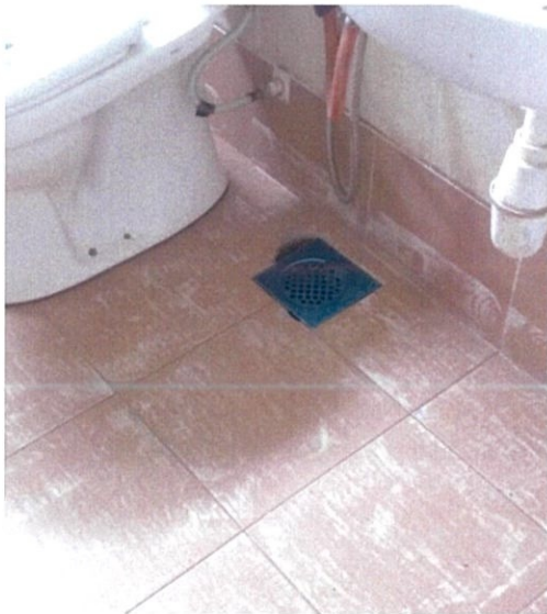
Figure 10 - Toilet are clean to provide a better epoxy condition.
