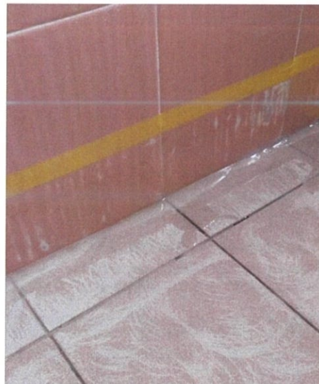
Figure 12 - Tape on top of 4 inches of skirting.
