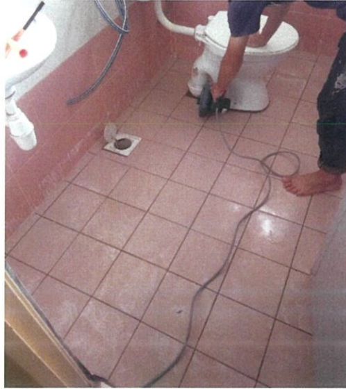
Figure 7 - Every corner need to be blow.
