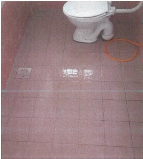
Figure 2 - Toilet's flooring need to be wash for the next step.
