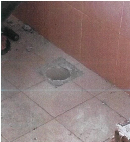
Figure 4 - Cement around the trap also need to be break.
