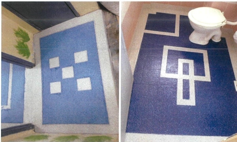
Figure 29 - Epoxy flooring finishing look.
