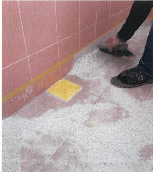
Figure 27 - Using broom to spread the flakes nicely.
