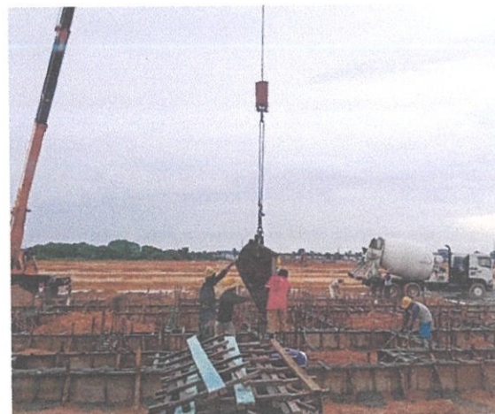
Figure 3.13 Pouring concrete for ground beam
