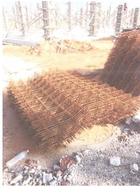
Figure 3.5 BRC for ground slab
