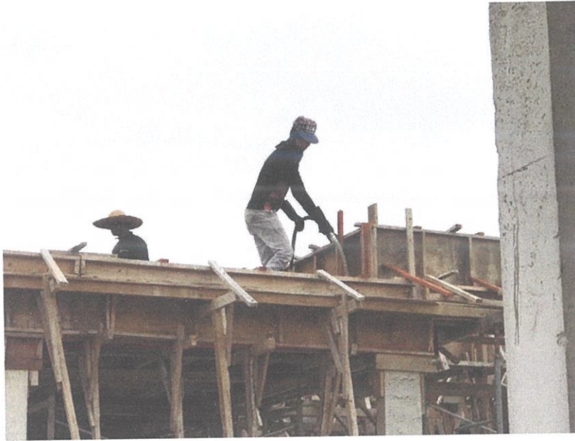
Figure 3.14 Concreter is compacting the concrete
