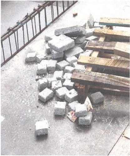
Figure 3.8 Concrete spacing blocks
