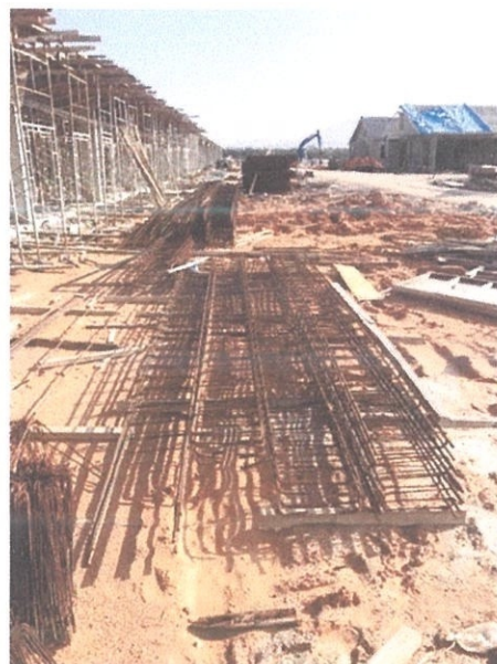
Figure 3.6 Reinforcement bars for column.
