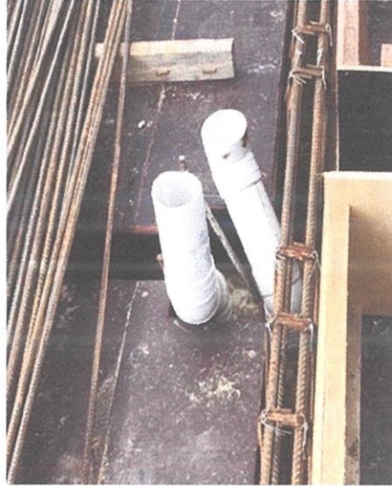
Figure 3.9 Installation of pipework
