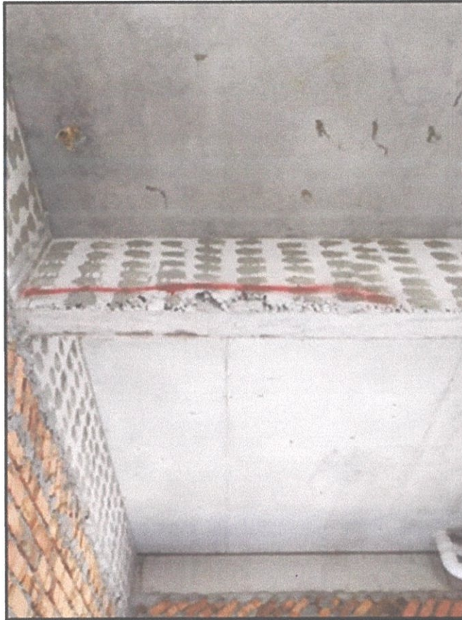
Figure 3.22 Honeycomb defect
