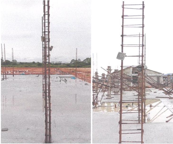
Figure 3.16 Inspection reinforcement bars before formwork
