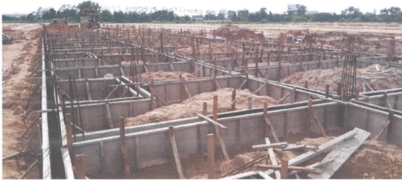
Figure 3.19 Installation formwork of ground beam
