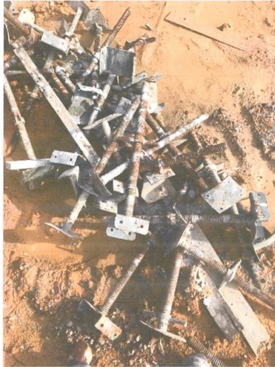
Figure 3.4 Braced for formwork
