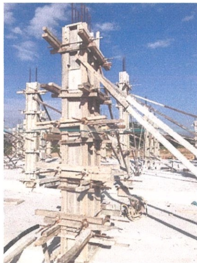
Figure 3.17 Inspection the vertically before concreting
