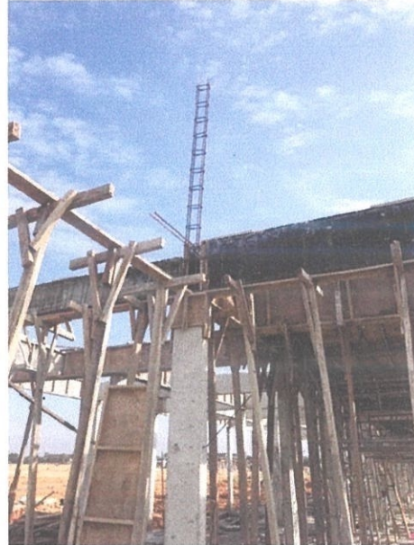
Figure 3.18 Formwork of beam
