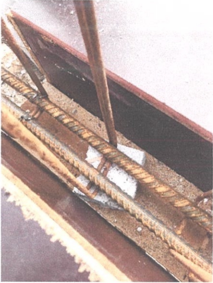
Figure 3.7 Installation of concrete spacing blocks
