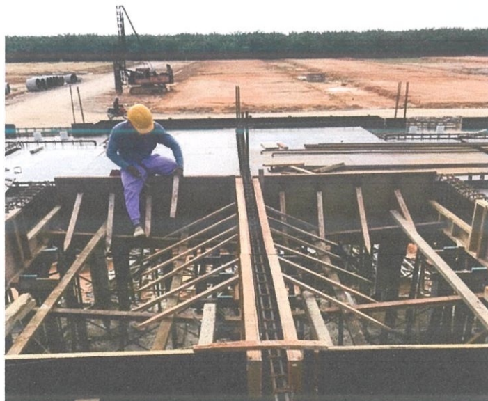
Figure 3.3 Installation of formwork
