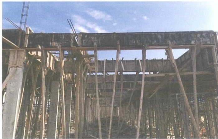
Figure 3.2 Design of formwork
