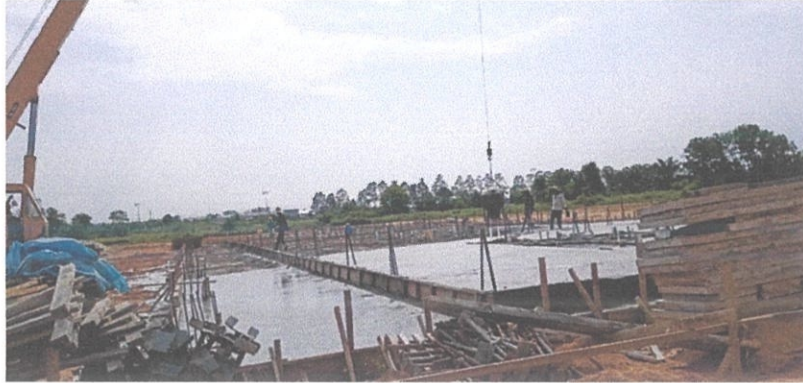
Figure 3.21 Pouring concrete for slab
