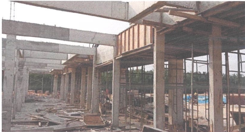
Figure 3.15 Stripping of formwork
