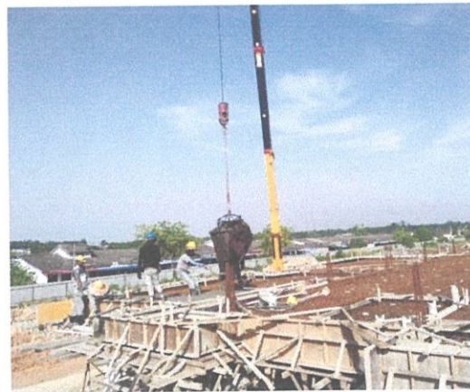
Figure 3.11 Pouring concrete for slab
