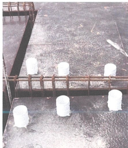
Figure 3.10 Installation of pipework
