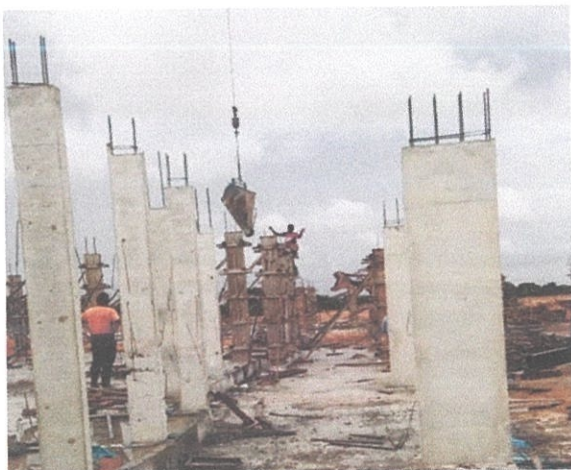
Figure 3.12 Pouring concrete for column
