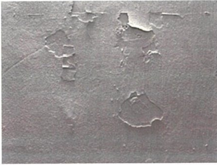
Figure 14.3.1: Peeling paint.
