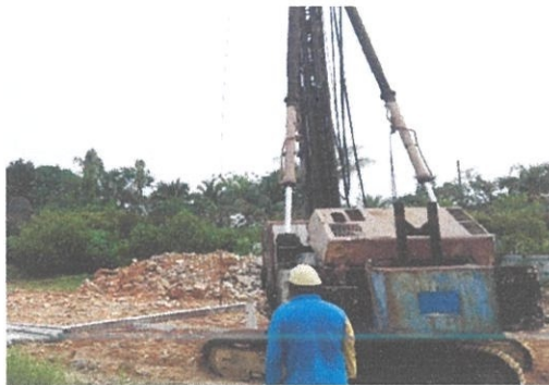
Figure 3.7: Pile Lifting into piling point
