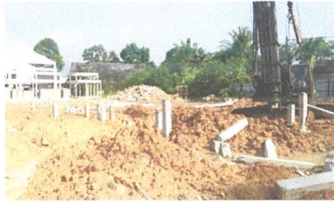
Figure 3.14 After Pile Process
