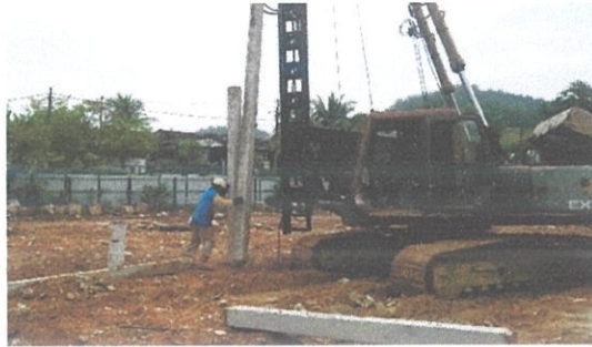
Figure 3.8 : Pile Positioning onto the piling point
