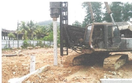
Figure 3.11: Hammering pile into ground
