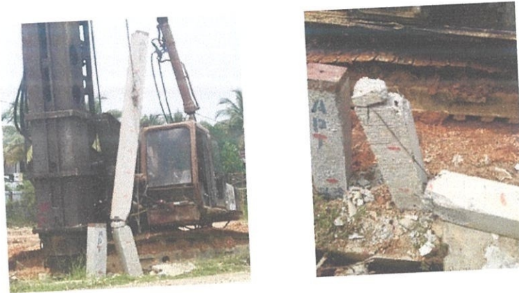
Figure 3.13 : Cracks Pile
