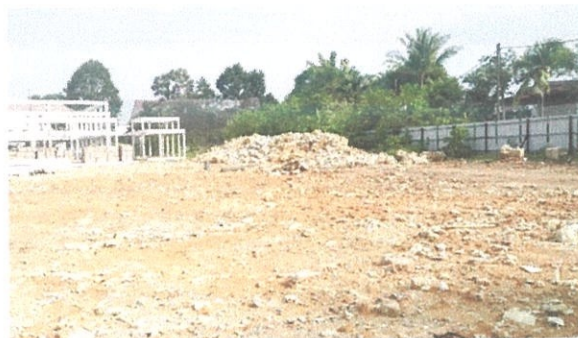
Figure 3.1: Location of piling work
