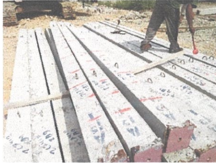
Figure 3.6 : Marking of concrete pile
