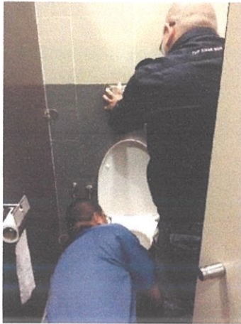
Photo 3. 2 The drainage is checked in the ladies' toilet no 2.
