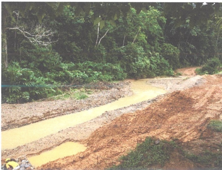
Figure 19: The River that been choose to construct gabion
