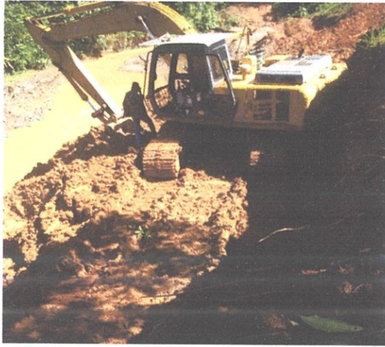
Figure 11: Base area of the cage was excavated using excavator
