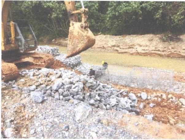
Figure 13: Filled up the rocks into the gabion cage
