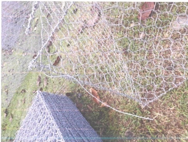
Figure 14: The cage was tied using steel wire
