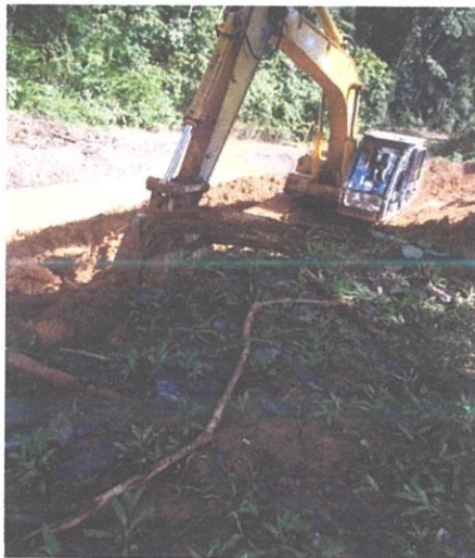
Figure 10: Clearance conducted by backhoe
