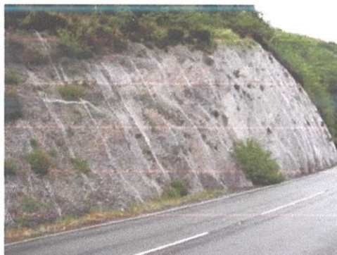
Figure 4: Shows the Gabion Wire Mesh
