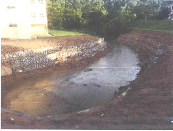
Figure 15: Gabion cage already installed at the side of the river
