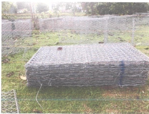
Figure 12: Gabion cage already installed
