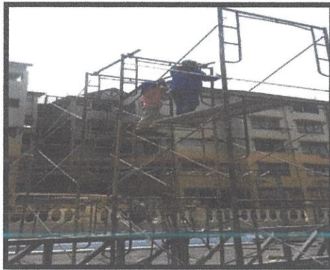
Figure 3. 36: Labor was lifting truss B using chain block.
