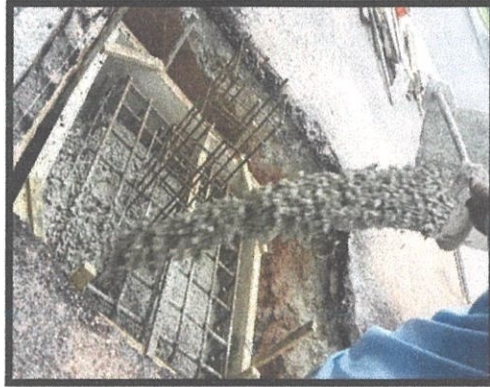
Figure 3. 25: Formwork were poured concrete.
