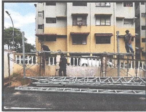
Figure 3. 31: Labors lifting truss on scaffolding.
