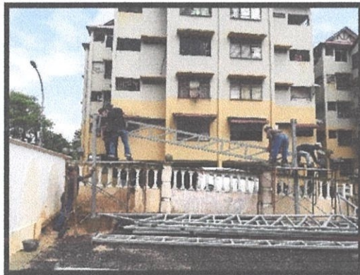
Figure 3. 32: Labor lifting truss on one side.
