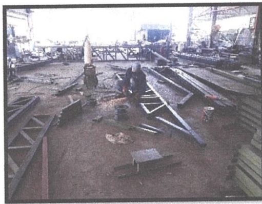
Figure 3. 8: Labor was grinding the excess material of welding.
