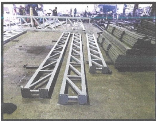
Figure 3. 17: Finished truss painting.
