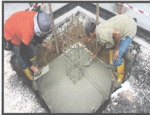
Figure 3. 26: Labors were rendering the concrete smooth.
