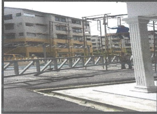
Figure 3. 35: Labor were lifting truss A using chain block.
