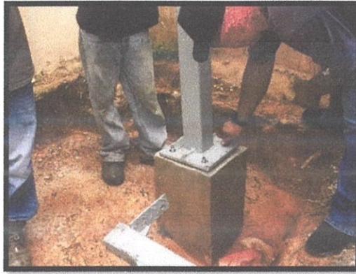
Figure 3. 29: Labors are lifting the steel column.
