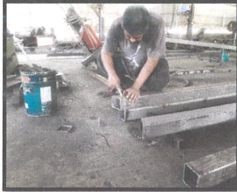
Figure 3. 18: Labor was measuring and marking the steel column.
