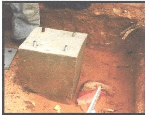
Figure 3. 28: Column stump after cured 3 days.
