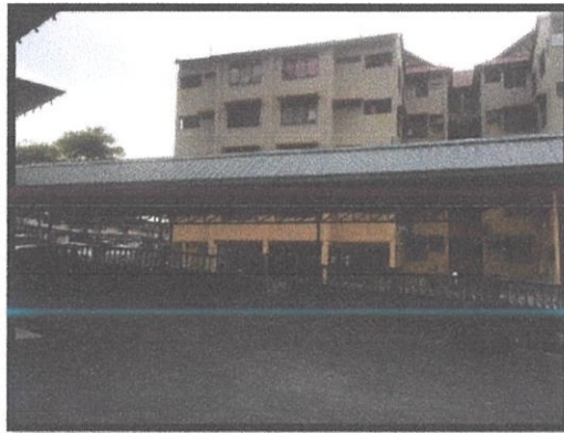
Figure 3. 38: Metal deck and gutter were installed.
