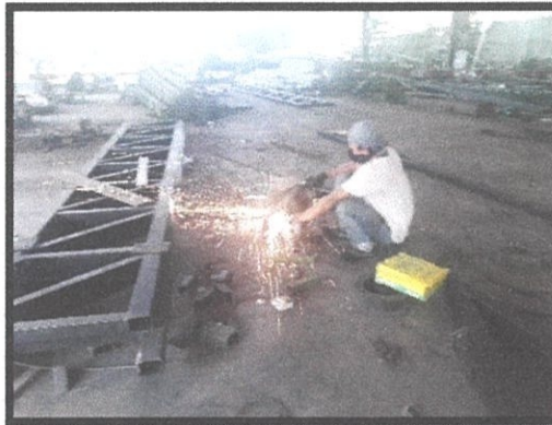
Figure 3. 4: Labor was cutting steel for frame.
