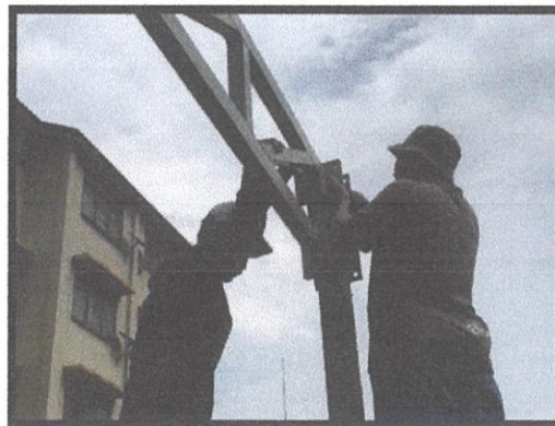
Figure 3. 34: Labors screwing bolt and nut at the plate.
