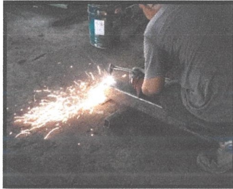
Figure 3. 19: Labor was cutting the steel column using oxy-acetylene cutting torch.
