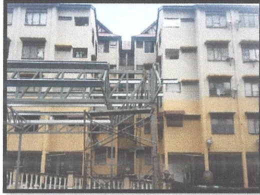
Figure 3. 37: Purlin were installed.
