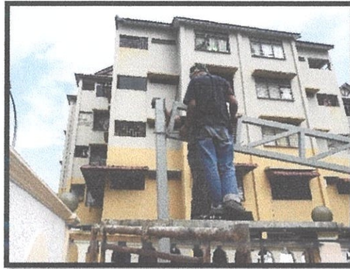
Figure 3. 33: Labor puts a round bar for temporary structure.
