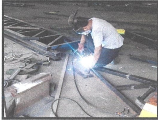
Figure 3. 5: Labor was fabricating the steel frame.
