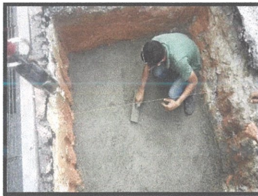
Figure 3. 22: Labor was rendering lean concrete smooth and evenly spread.
