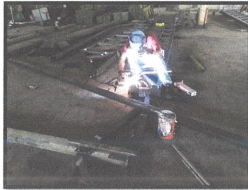
Figure 3. 13: Labor fabricating with 6mm thick fillet weld.
