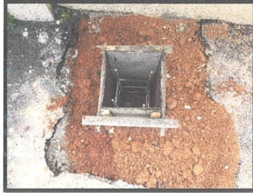
Figure 3. 27: Formwork of column stump
