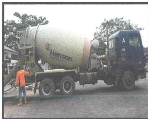
Figure 3. 24: Cement mixer truck was arrived at site.
