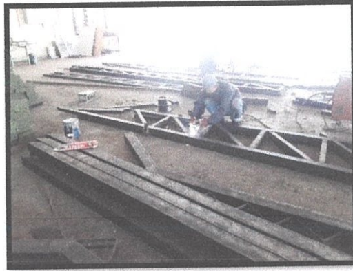
Figure 3. 7: Labor fabricating struts and diagonal to the frame of truss.
