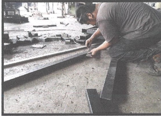
Figure 3. 3: Labor marking the excess steel.
