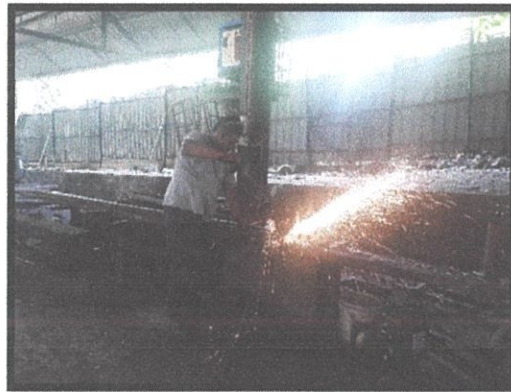
Figure 3. 6: Labor was cutting steel for strut and diagonal members.
