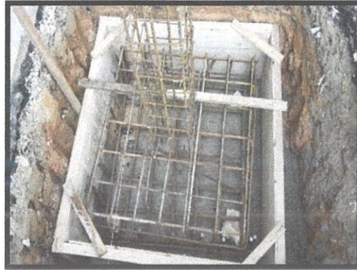
Figure 3. 23: Formwork and reinforcement bar.
