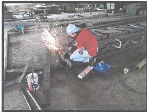
Figure 3. 14: Labor was grinding the excess material.
