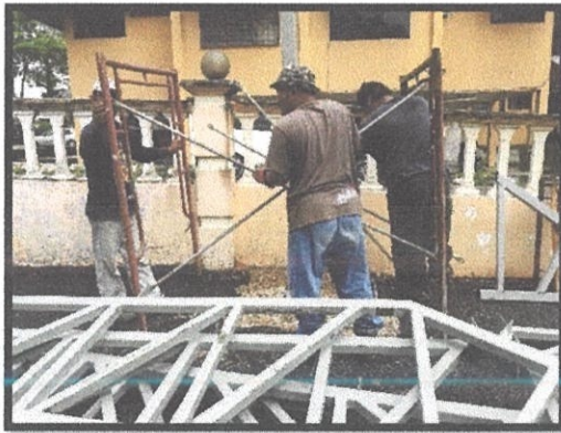
Figure 3. 30: Labor were erecting scaffolding.
