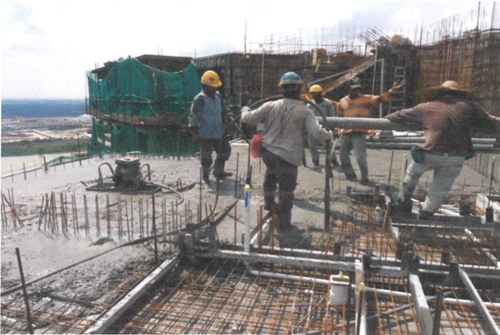
Figure 3.11 compaction of concrete process
