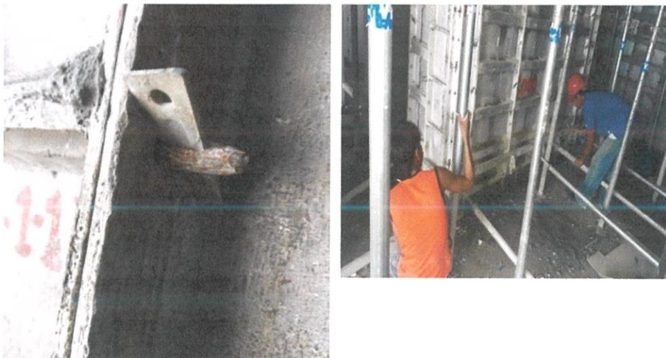
Figure 3.9 Checking for formwork tightness
