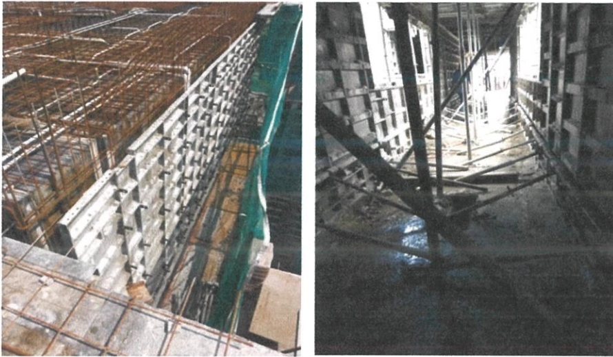
Figure 3.8 Installed formwork and shoring
