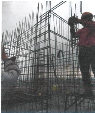
Figure 3.10 Insertion of spacer block and tying reinforcement bars
