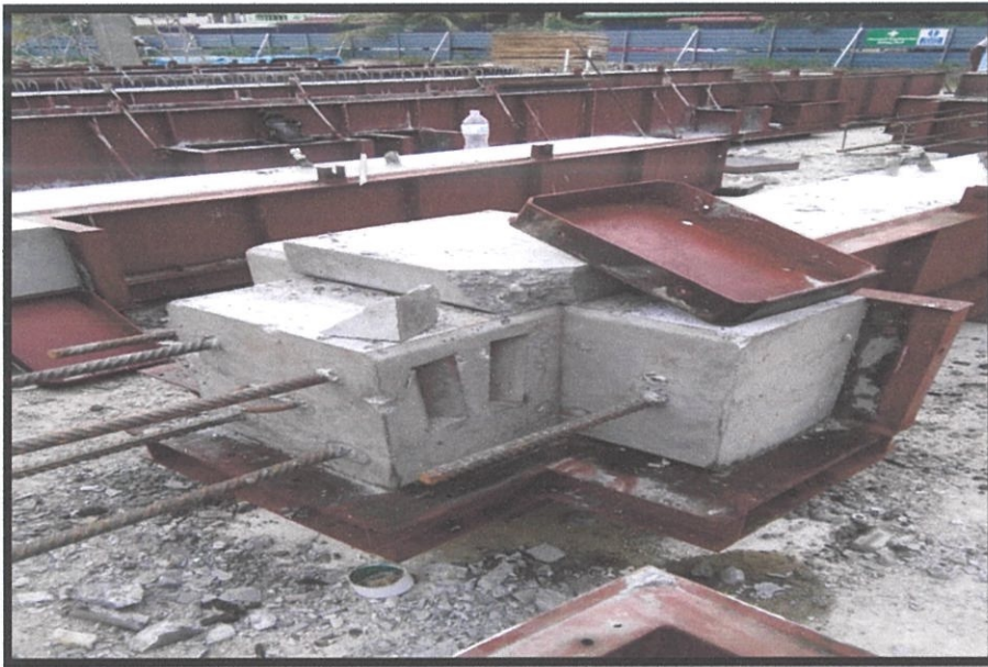
Figure 3.11: The de-moulding of precast column from steel mould
