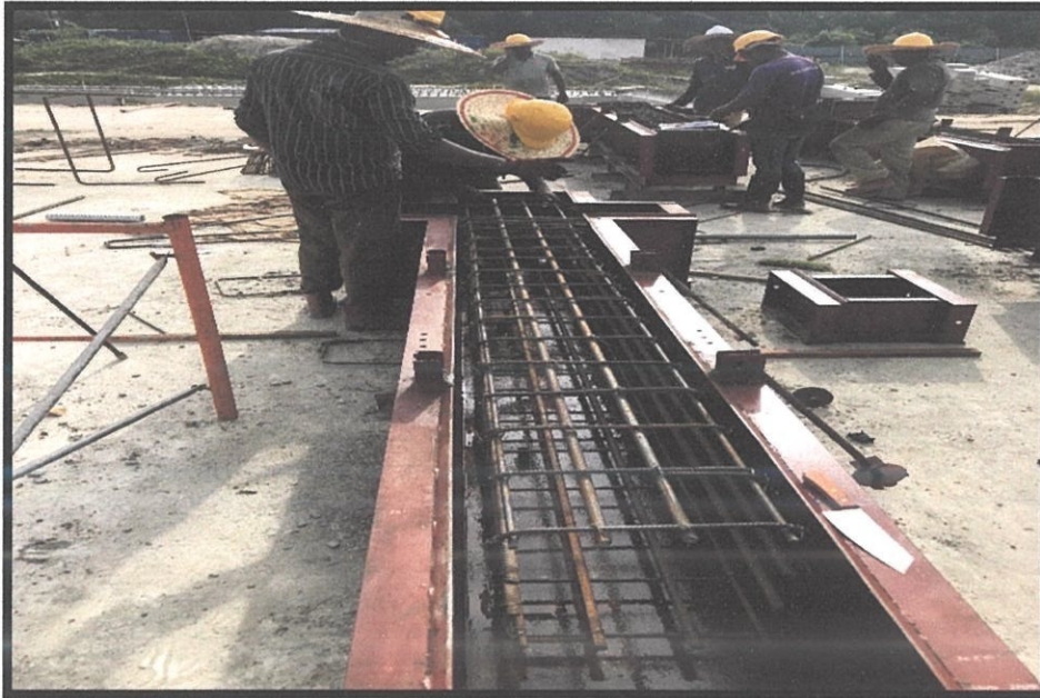
Figure 3.9: The fixing of reinforcements inside mould
