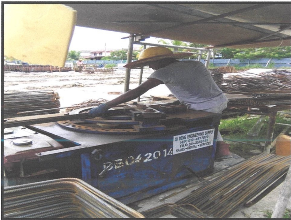
Figure 3.8: The bending of reinforcement bars by barbender
