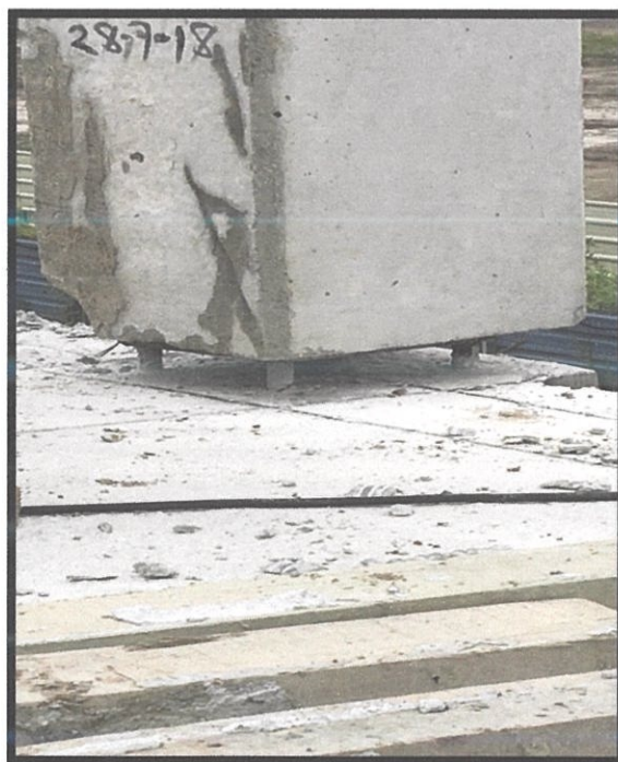
Figure 3.14: The precast column that has been marked.
