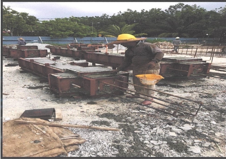
Figure 3.6: Precast reinforced concrete products cast in steel moulds
