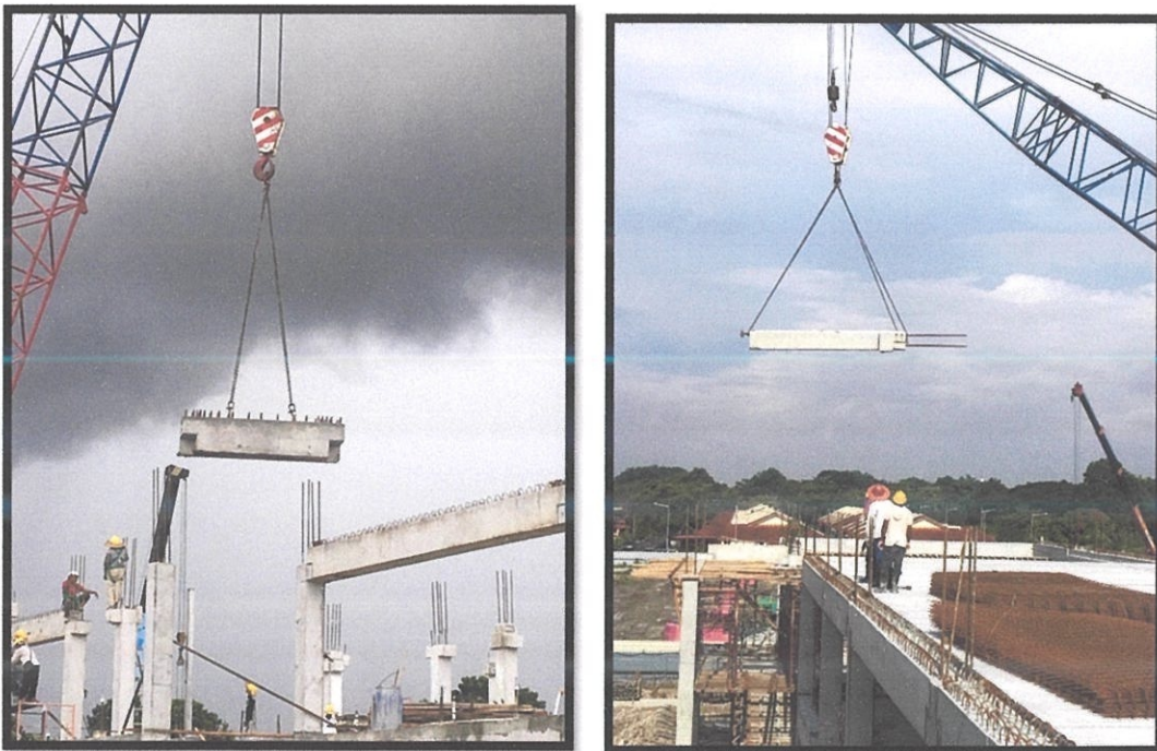
Figure 3.12: The lifting of beam and column using a crawler crane
