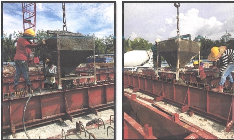
Figure 3.7: The process of mixing concrete poured into the steel moulds
