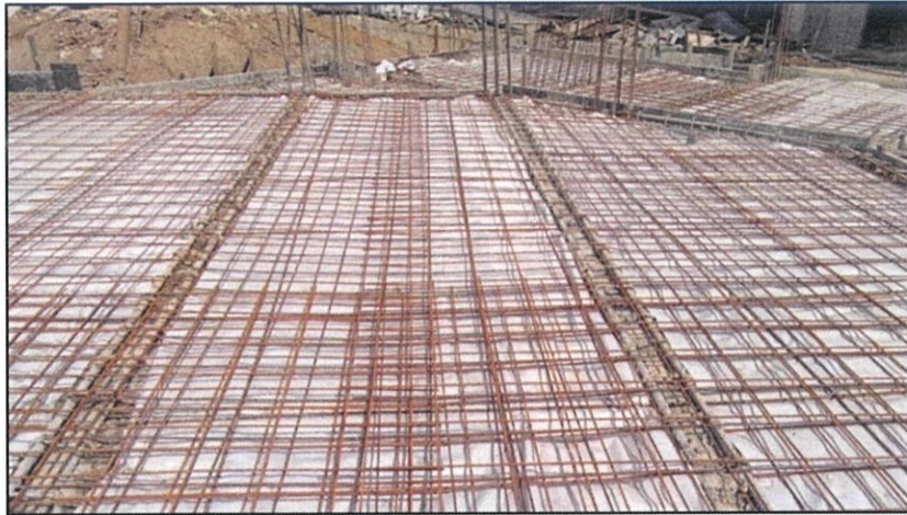
Photo 3.26 BRC has been used at construction site
