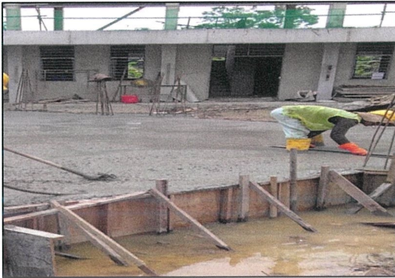
Photo 3.16 Skilled labour screeding the top of concrete
