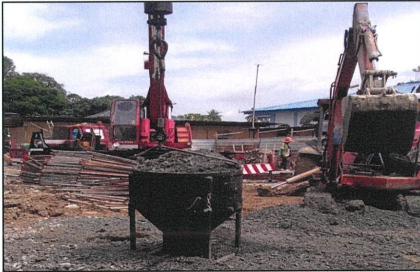
Photo 3.5 The backhoe filling the gravel into concrete bucket
