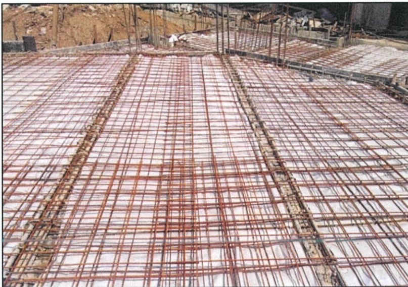
Photo 3.10 BRC has been installed by skilled labours.
