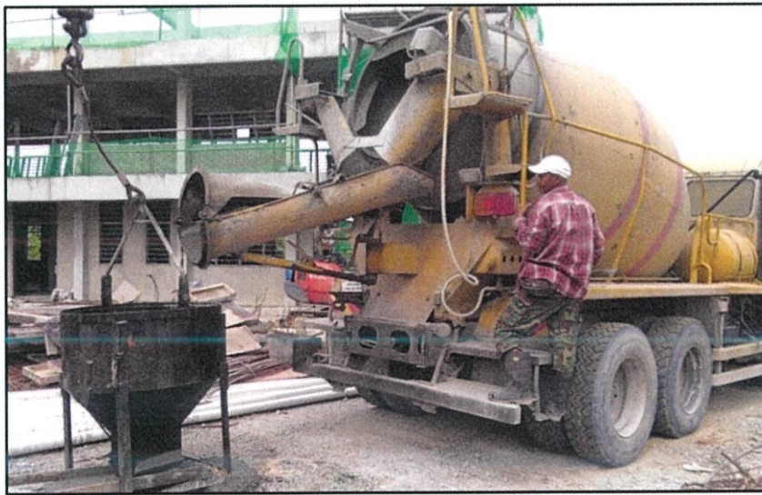
Photo 3.13 Fresh concrete was poured into the concrete bucket.
