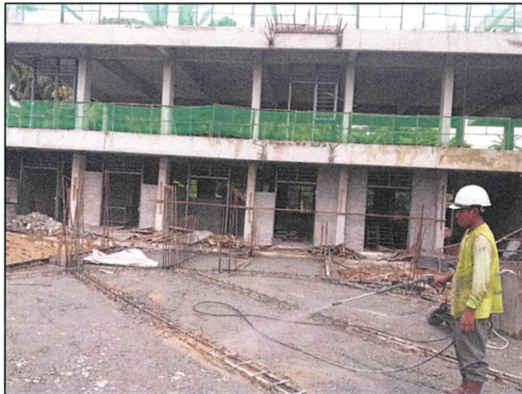
Photo 3.8 skilled labour spray anti-termite
