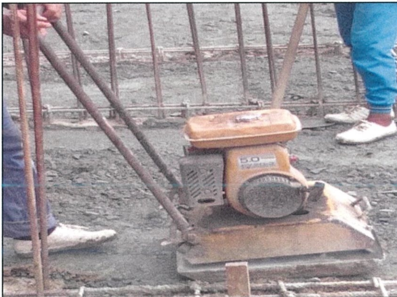
Photo 3.23 Plate compactor machine
