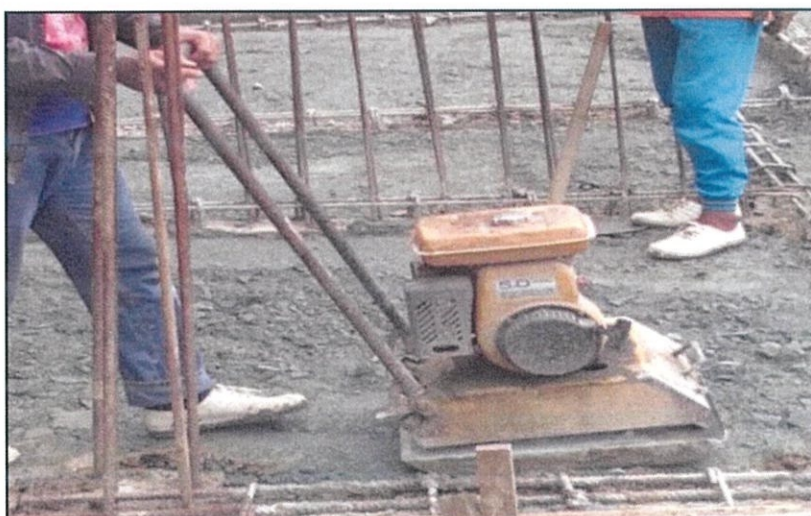
Photo 3.7 Plate compactor machine to compact the soil
