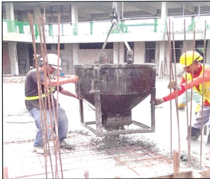
Photo 3.14 Fresh concrete was poured.
