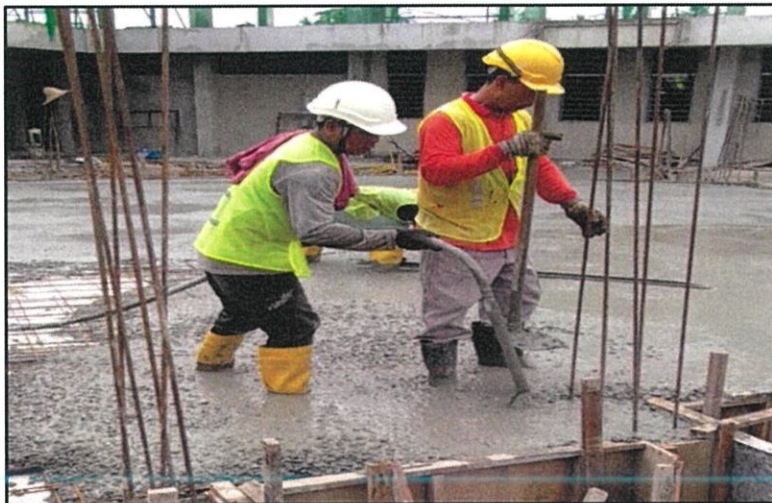
Photo 3.15 Skilled labour vibrating the concrete
