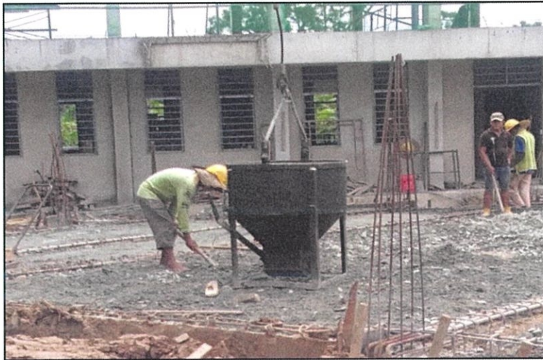
Photo 3.6 Skilled labour poured the gravel above the ground
