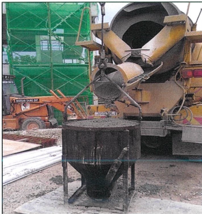
Photo 3.22 Concrete bucket
