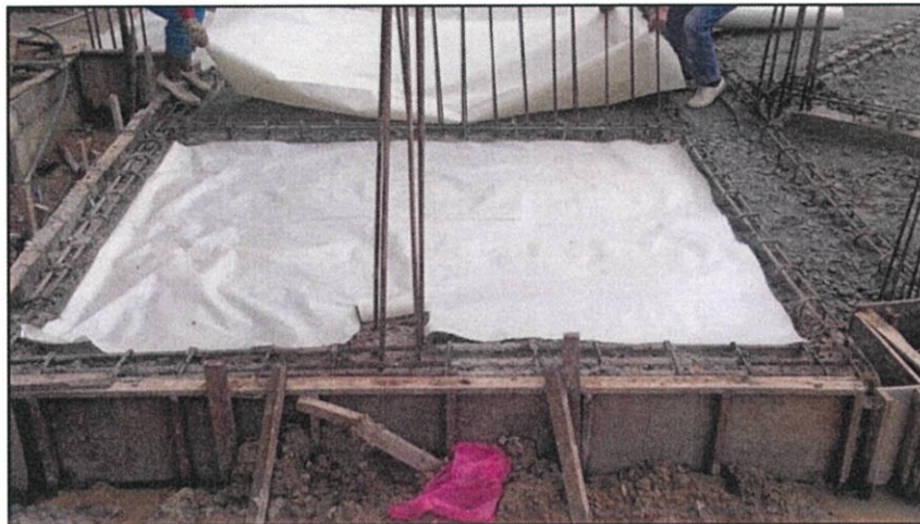
Photo 3.27 Polythene covering sheet as DPM
