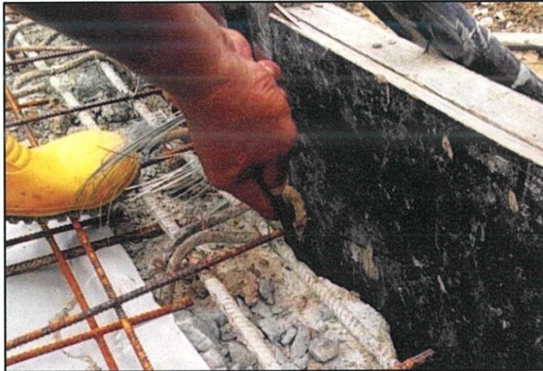
Photo 3.11 Skilled labour tying mesh wire on BRC
