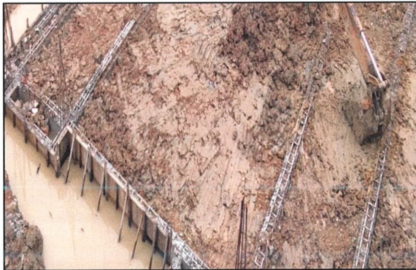
Photo 3.3 Ground beam has been completed from top view
