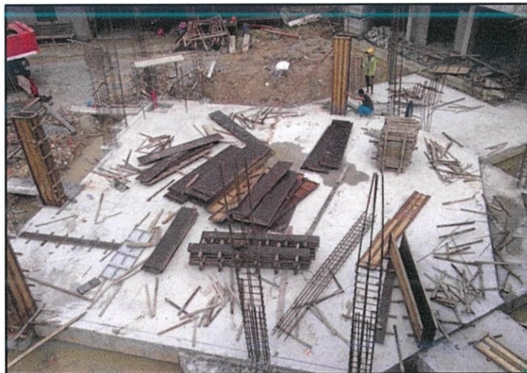
Photo 3.17 Formwork has been removed
