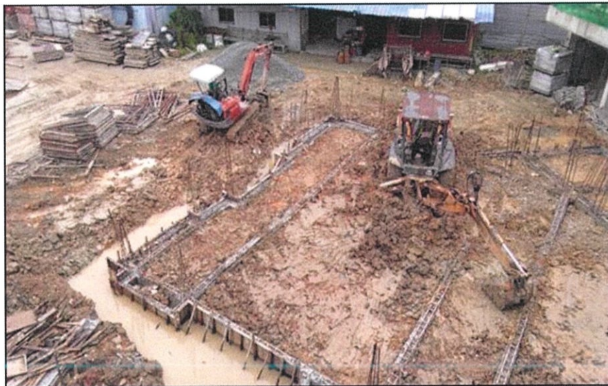
Photo 3.4 Excavator and backhoe operators doing excavating and backfilling soil work
