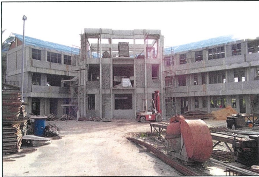
Photo 3.1 Front elevation of the site project
