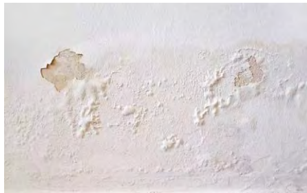
Figure 1: Peeling paint
