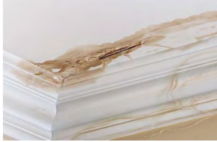
Figure 2: Roof leakage
