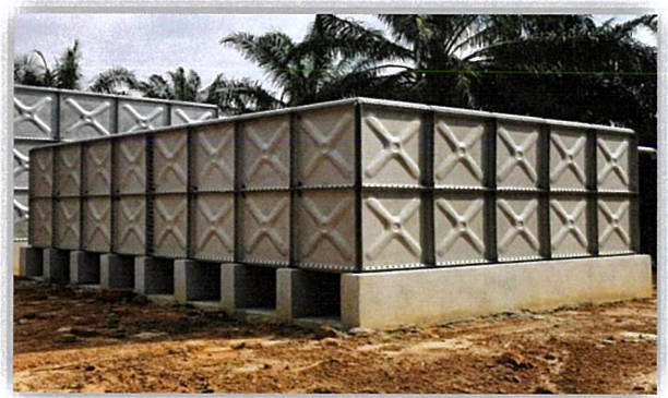
Figure 3 : Stainless Steel Water Tank
