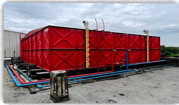
Figure 2 : Pressed Steel Water Tank
