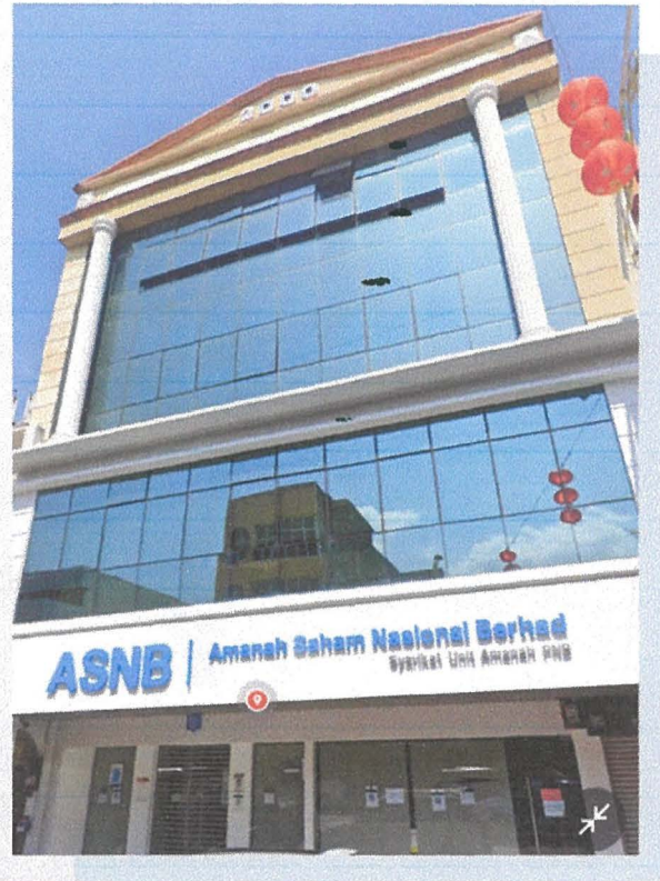
Figure 6: ASNB Seremban Branch
