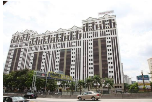
Figure 3 Synergy Group Damansara Intan
