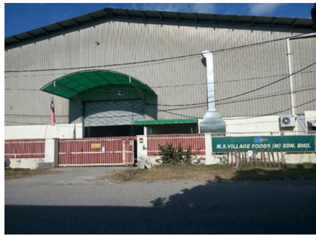
Figure 10.2: Front view of company
