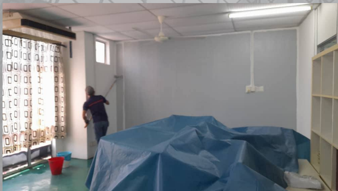
Monitor the office renovation.
