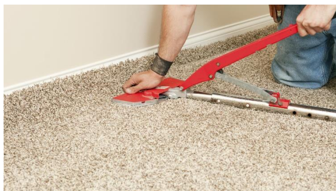
Figure 2.5 Pressing down the carpet
