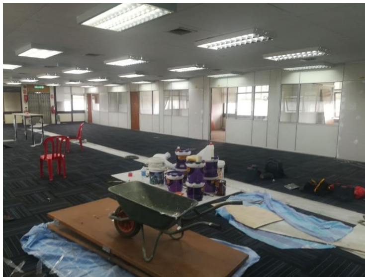
Figure 2.3 Office condition during renovation
