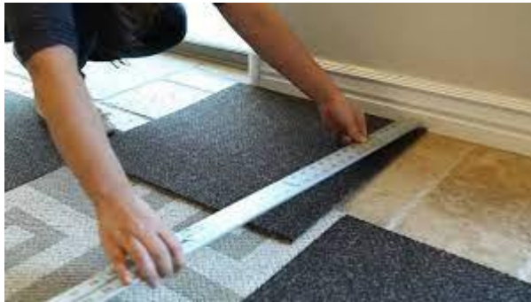
Figure 2.4 Measuring size of carpet
