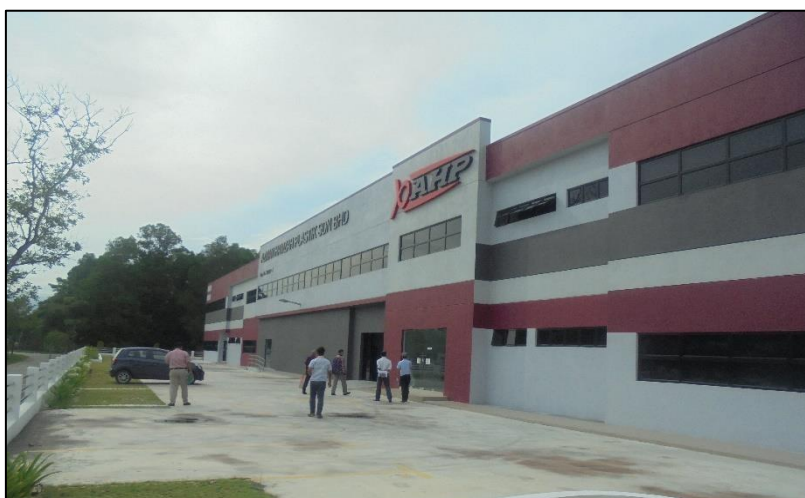
Figure 3.5 : View of the case study.
