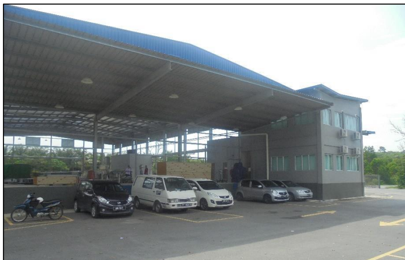
Figure 3.9 : View of the case study.
