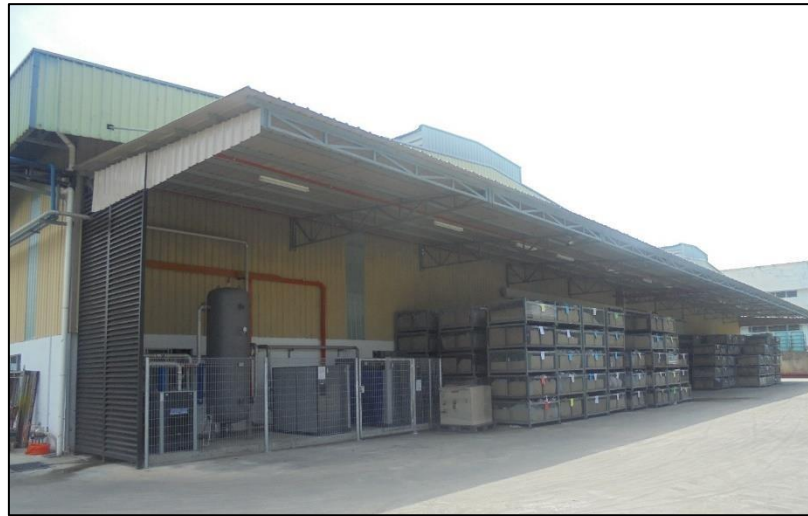
Figure 3.14 : View of the case study.
