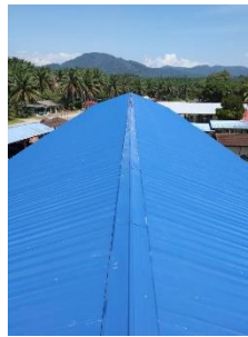
Figure 26 Installing of New Metal Deck Rafters
