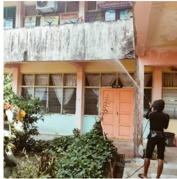
Figure 37: Water Jet to Remove
