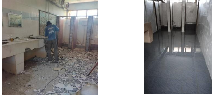
Figure 29: New laid tiles at the affected areas in the toilet.
