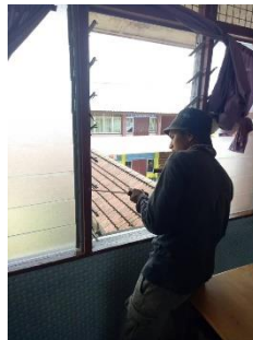
Figure 34: Newly Installed of Nako mirror
