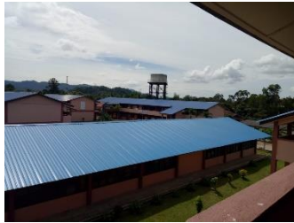
Figure 25: Installation of New Metal Deck Roof
