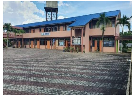
Figure 24: Newly Installed of Roof
