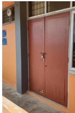
Figure 32: Newly Installed Two Lead Wooden Door
