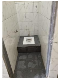
Figure 30: Installation of Toilet Bowl
