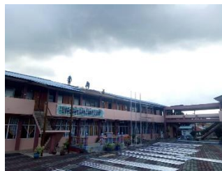
Figure 36: Installation of New Roof
