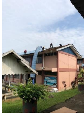
Figure 31: Installation of New Roof
