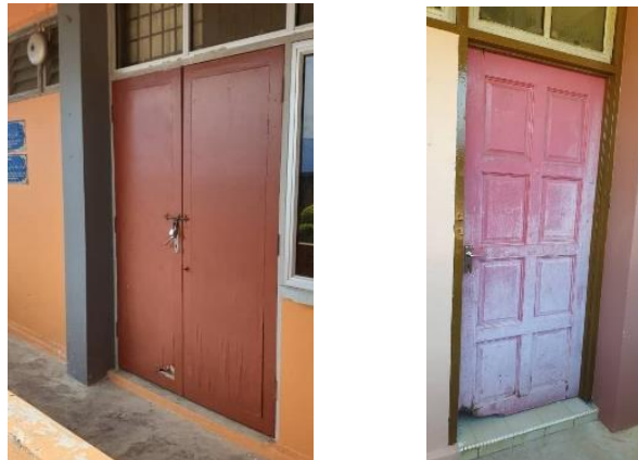
Figure 27: Newly Installed Single Lead and Two Lead Wooden Door
