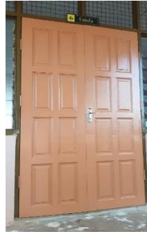
Figure 33: Newly Installed Two Leaf Solid Wood Door
