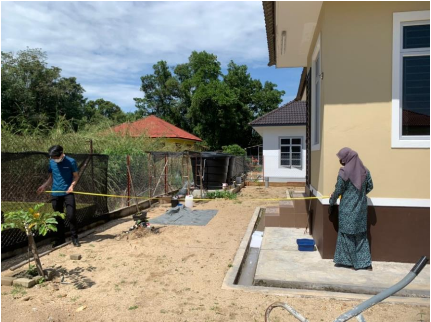
Figure 3.18 Shown measuring the house setback
