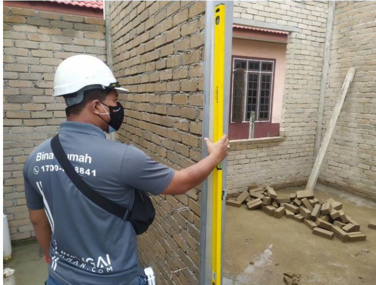
Figure 3.6 Site supervisor inspecting the construction site
