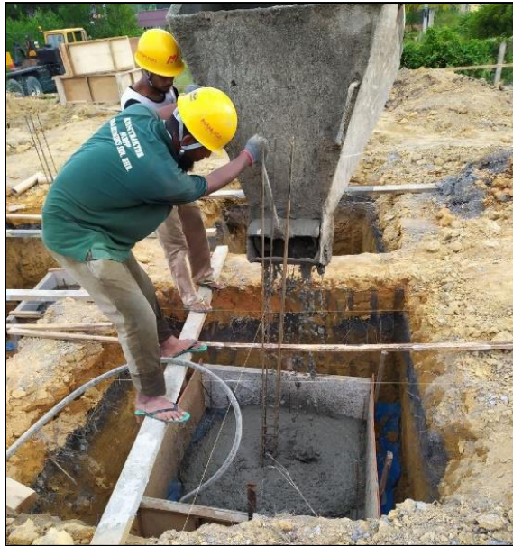
Figure 3.12 Semi-Skilled Workers Doing Concreting Works
