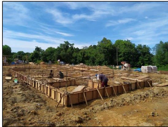
Figure 3.11 Semi-Skilled Workers Doing Formwork
