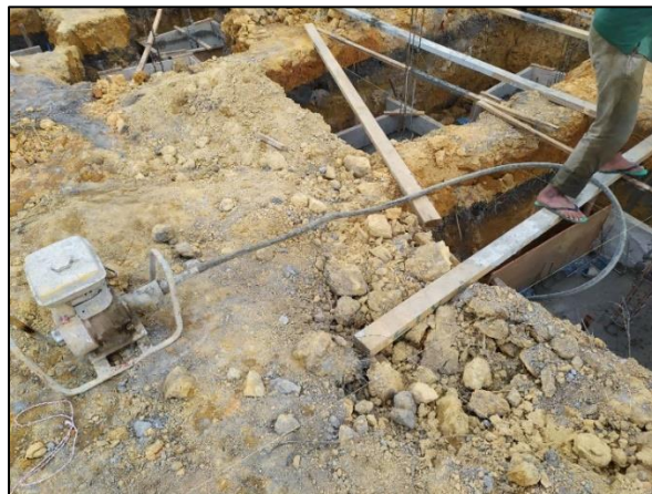
Figure 3.13 Semi-Skilled Workers Doing Concreting Works
