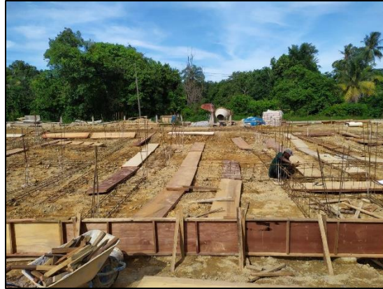
Figure 3.10 Skilled Workers Doing Formwork
