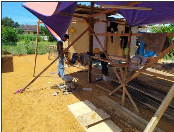
Figure 3.9 Semi-Skilled Workers Doing Steelworks
