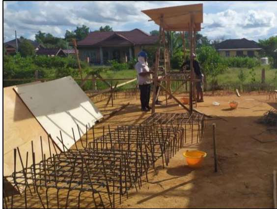
Figure 3.8 Skilled Workers Doing Steelworks
