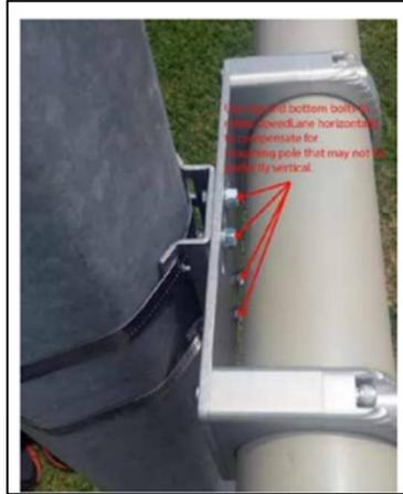
**Figure 6.** Installation of the mounting bracket (Houston Radar, 2018).
