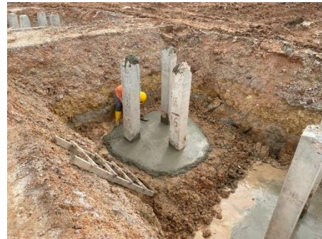
Figure 3.21 : Laying lean concrete
