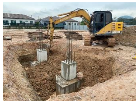
Figure 3.31 : Backfilling
