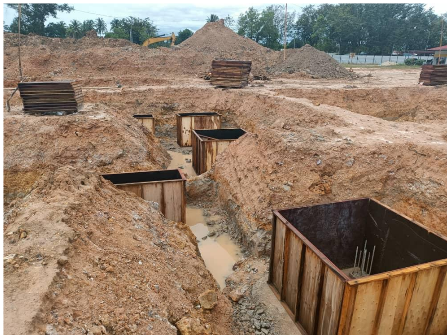
Figure 3.15 : Pile cap formwork
