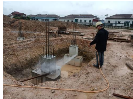
Figure 3.30 : Applying anti termite on pile cap
