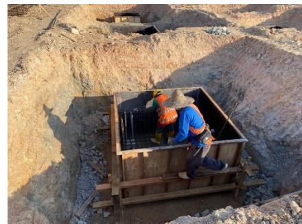
Figure 3.25 : Rebar installation
