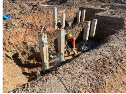
Figure 3.20 : Cutting pile works
