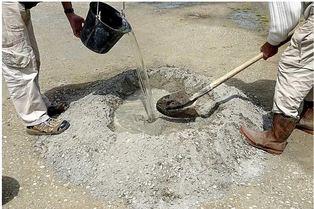
Figure 3.12 : The concrete mixture was mixed with water.
