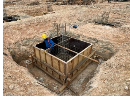
Figure 3.26 : Pile cap and rebar installation
