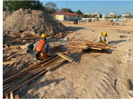
Figure 3.22 : Formwork for pile cap
