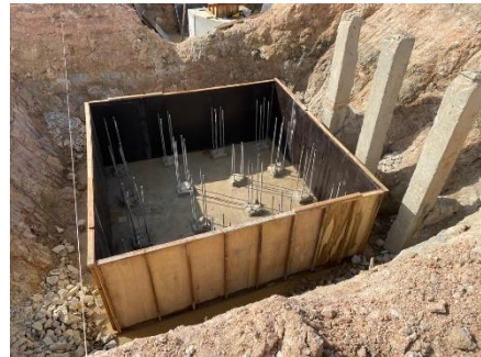
Figure 3.23 : Pile cap formwork
