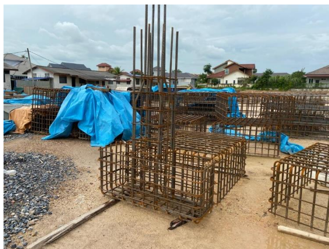
Figure 3.8 : Pile cap rebar
