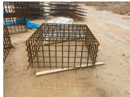
Figure 3.24 : Pile cap rebar
