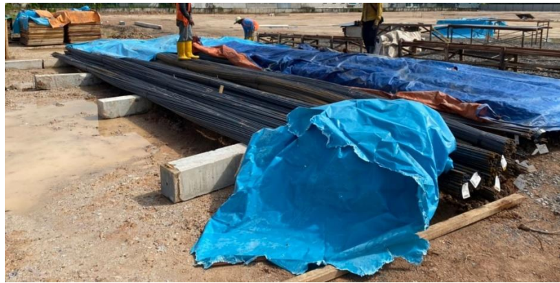
Figure 3.7 : Reinforcement steel bars
