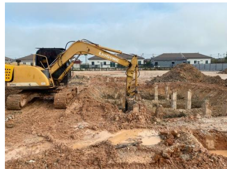
Figure 3.19 : Pile cap excavation
