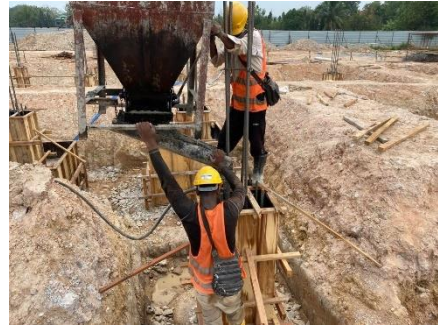
Figure 3.28 : Concreting work
