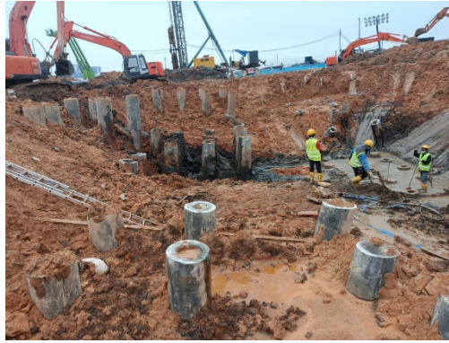
Figure 2.0 The Construction Progress of Pre-cast Concrete
