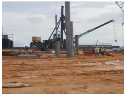
Figure 13.0 After Installation Pre-cast Concrete Piling by Injection Machine
