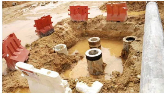
Figure 17.0 Pile Head Repaired
