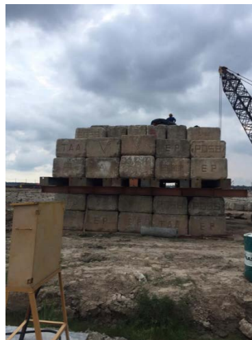
Figure 29.0 The Load Test
