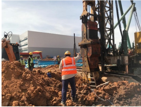
Figure 32.0 The setting of PDA Test
