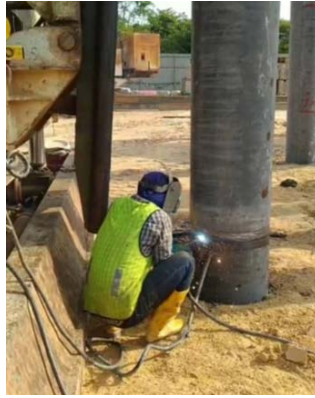
Figure 14.0 Pre-Cast Concrete Welding Process
