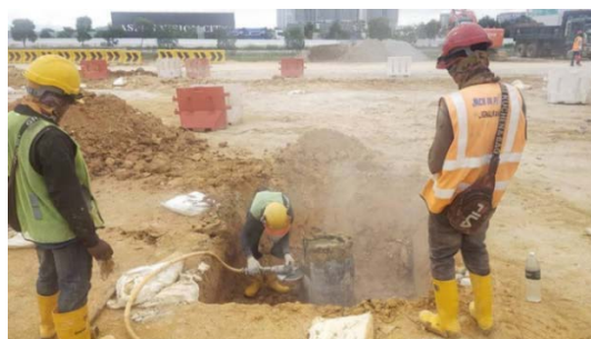
Figure 16.0 Pre-Cast Concrete Cutting Process
