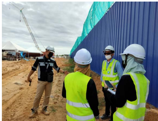
Figure 11.0 Site Visit with Site Manager
