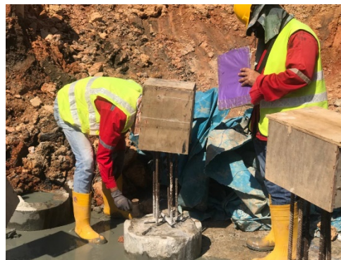
Figure 35.0 Geophone Placed on The Top of Pile
