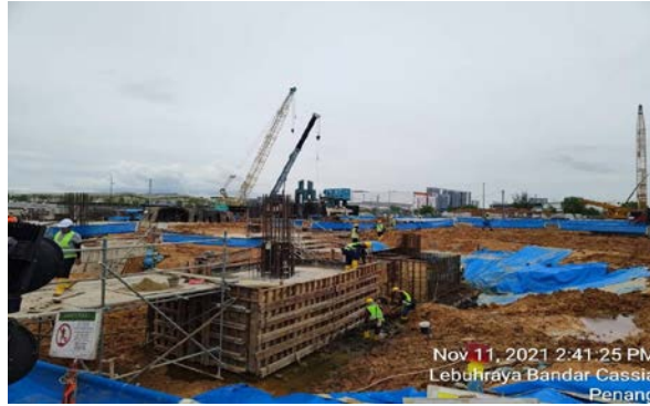
Figure 23.0 Formwork Installation
