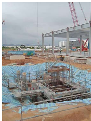
Figure 24.0 Concreting of The Pile Cap
