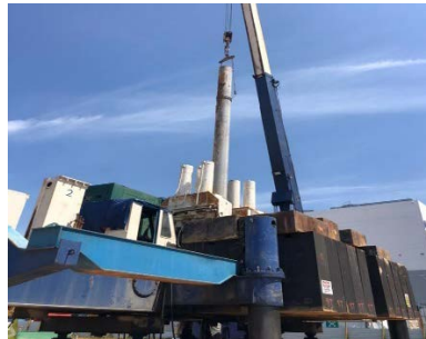
Figure 12.0 Pre-cast Concrete Piling Process Using Injection Machine
