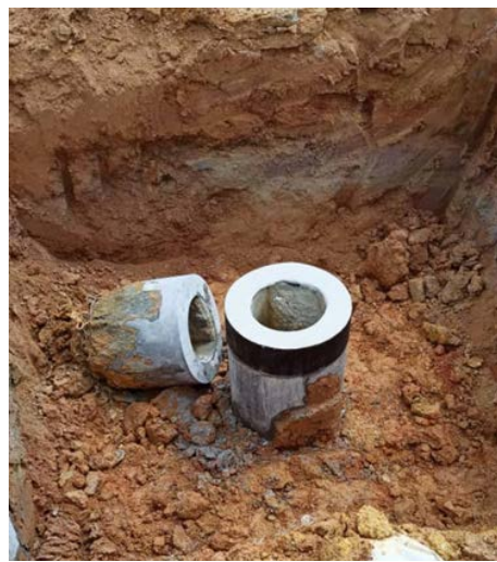
Figure 18.0 Pile Head after Repaired
