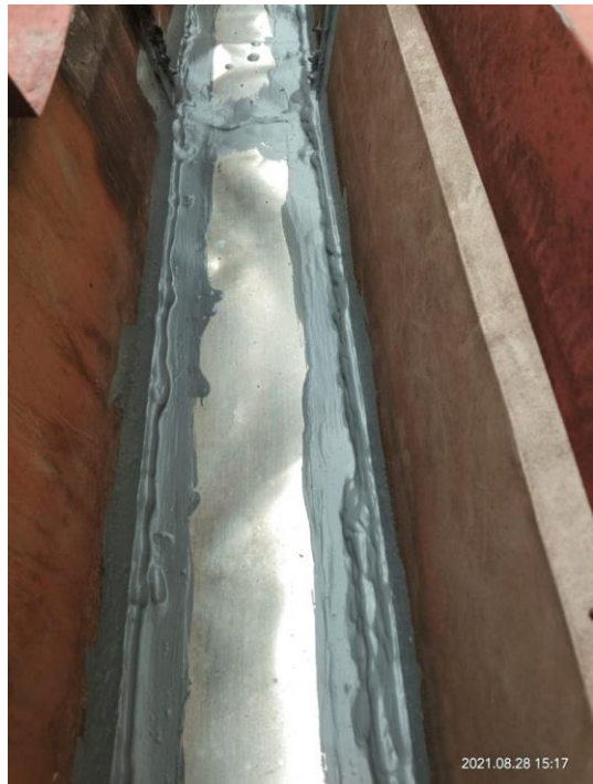
Figure 14: The gutter that has been attached with waterproofing tape and silicone
