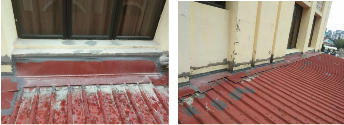
Figure 15: Flushing roof that has been installed
