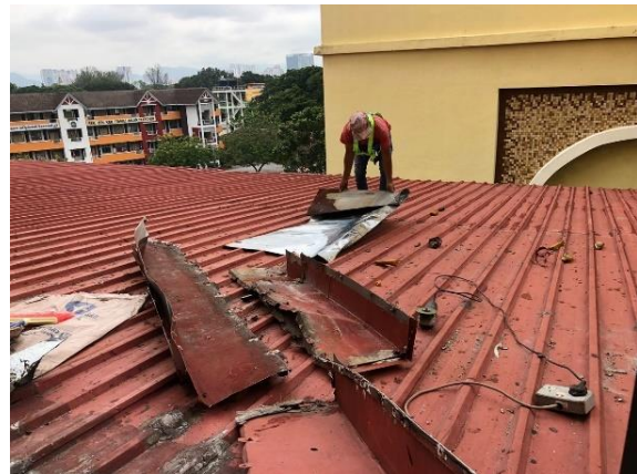
Figure 8: The flushing roof that had been removed
