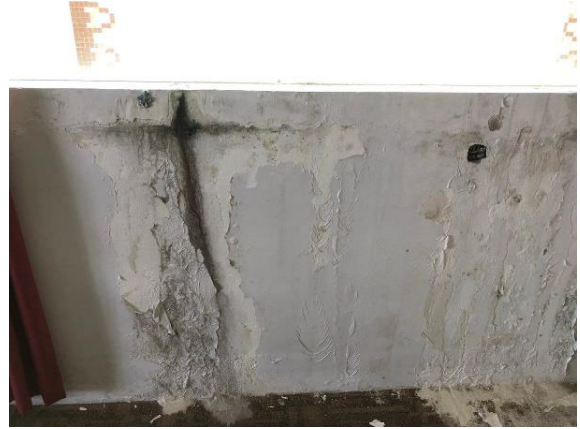
Figure 9: The wall that have damaged due to leakage
