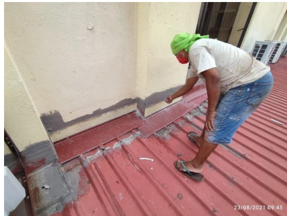
Figure 25: A roofing professional has completed the flashing roof installation work
