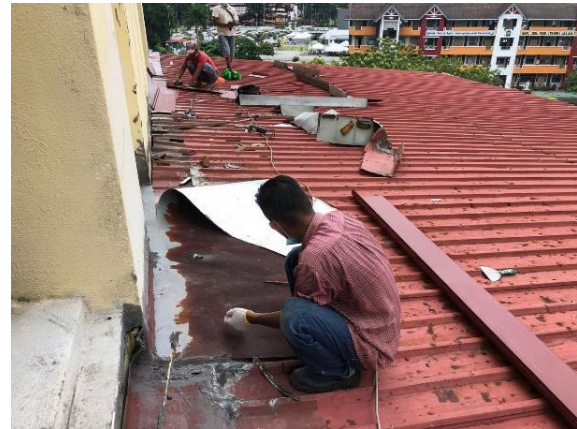
Figure 7: The workers are removing the air conditioner outdoor unit and flushing roof
