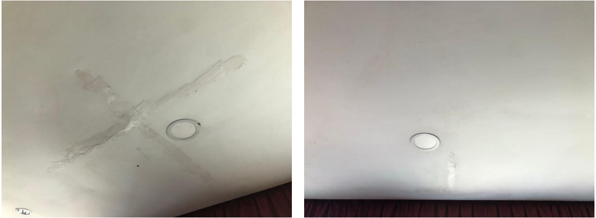
Figure 19: The ceilings that has been sealed and repainted
