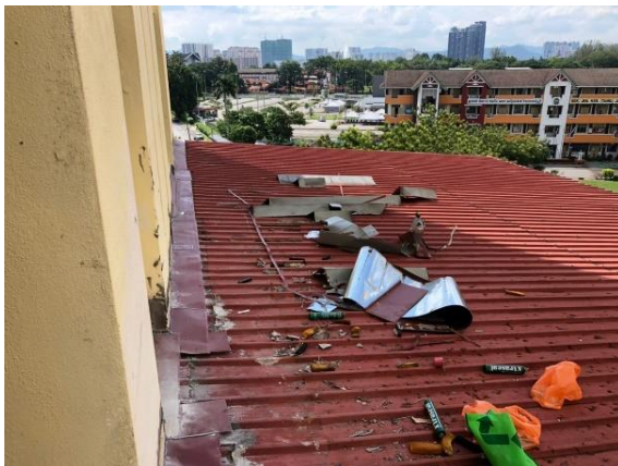
Figure 8: The flushing roof that had been removed
