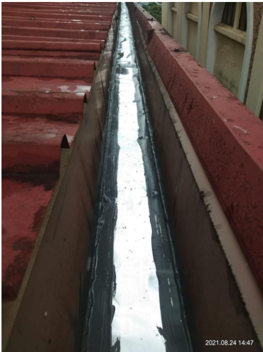
Figure 14: The gutter that has been attached with waterproofing tape and silicone
