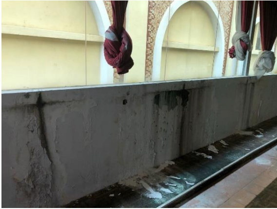
Figure 9: The wall that have damaged due to leakage
