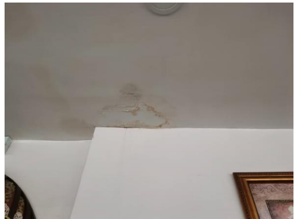
Figure 10: The damaged ceiling due to leakage
