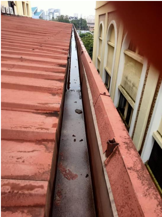
Figure 13: The gutter that has been cleaned and workers attached the waterproofing tape and silicone
