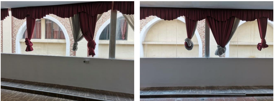
Figure 20: The walls that has been repainted
