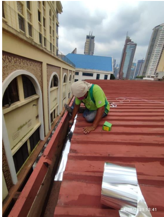
Figure 13: The gutter that has been cleaned and workers attached the waterproofing tape and silicone
