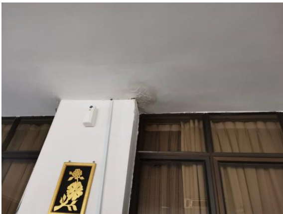
Figure 10: The damaged ceiling due to leakage
