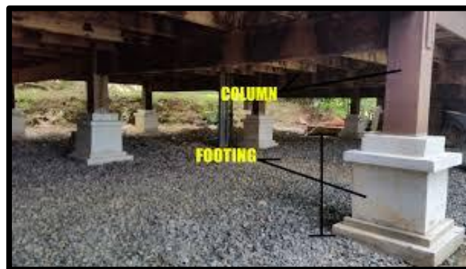
Figure 2.4.3: Base of The Column
