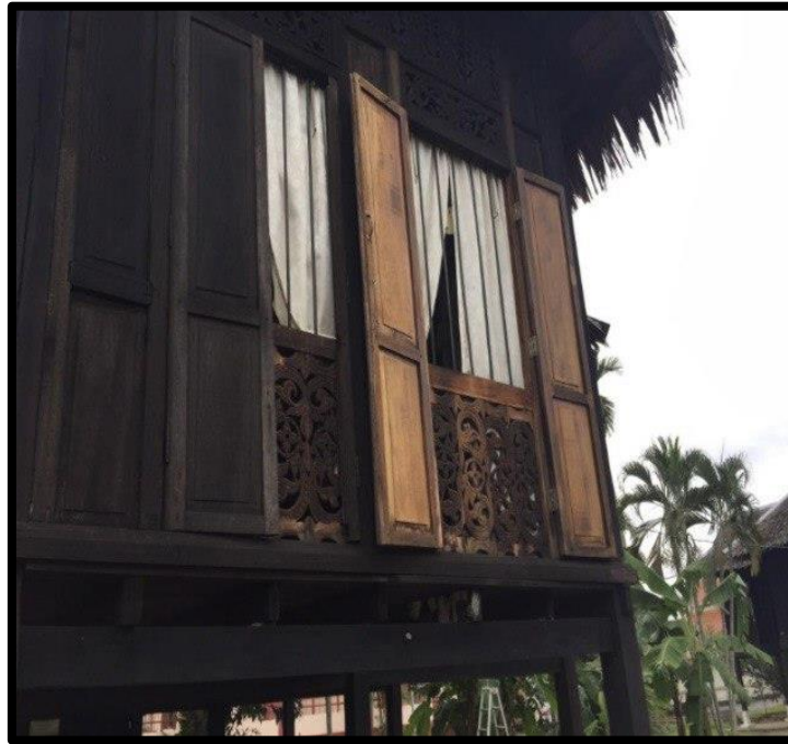
Figure 3.4.3.1: Double Casement Windows
