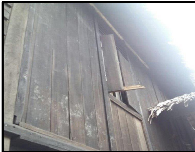
Figure 4.1.4.1: Window Defect
