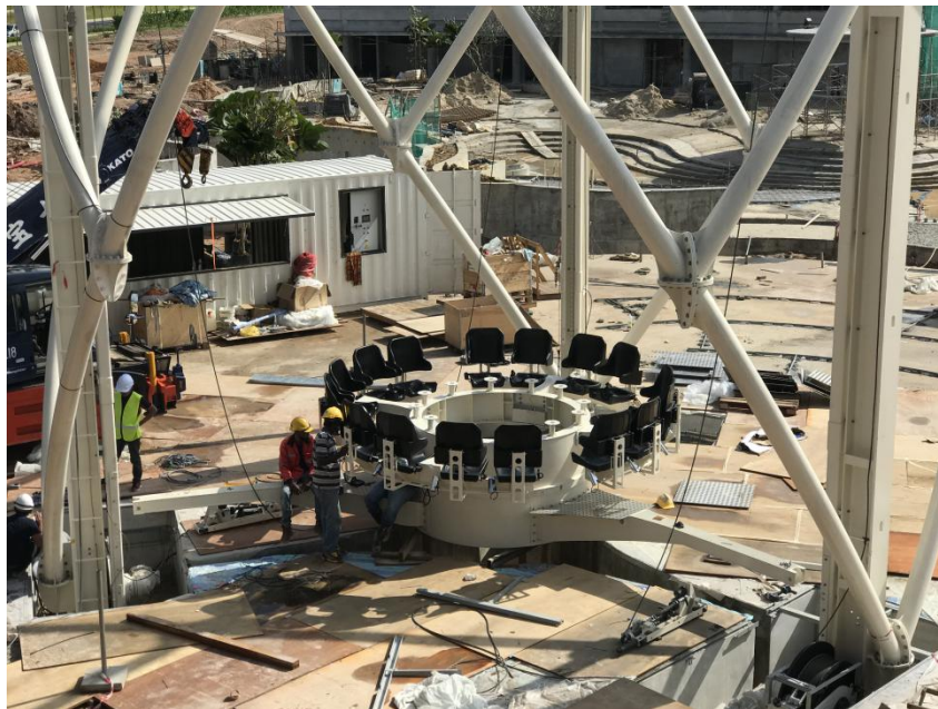
Figure 8: Construction of Aerobar.
