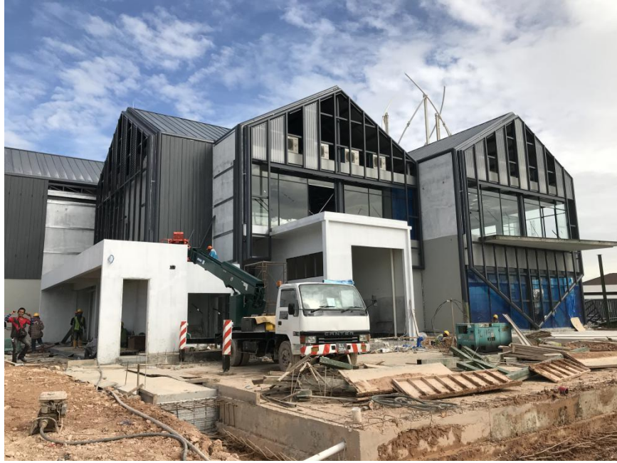
Figure 9: Construction of retail building.
