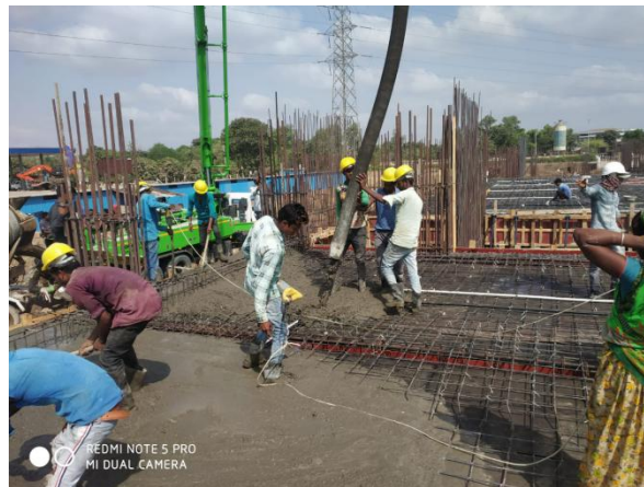
Figure 2: Cast In-situ concrete slab.
