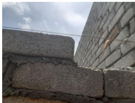
Figure 3.2.4: Strings that pinned together in between column.
