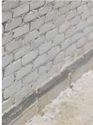
Figure 3.2.5 Installed Damp Proof Course above the floor surface for the wall.
