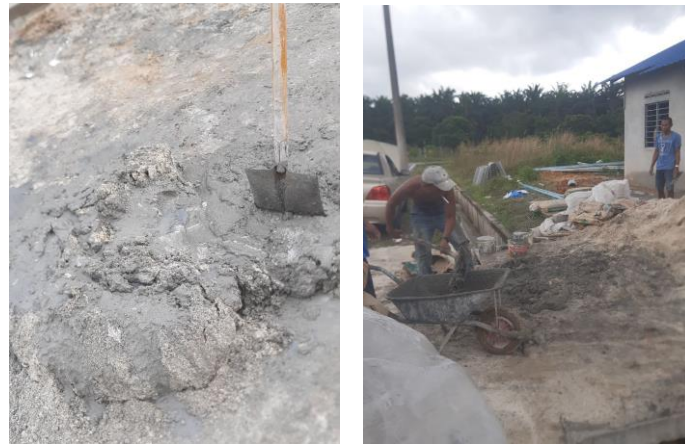
Figure 3.2.3: Mortar are mixed manually.
