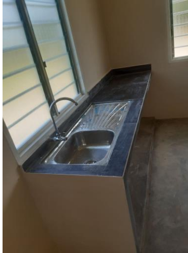
Figure 3.3.11 the picture show after brickwork process for table top
