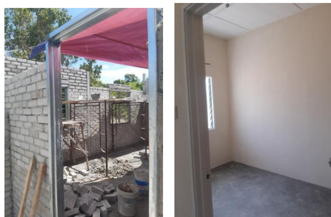
Figure 3.3.8 the picture show before and after brickwork process for bedroom 3
