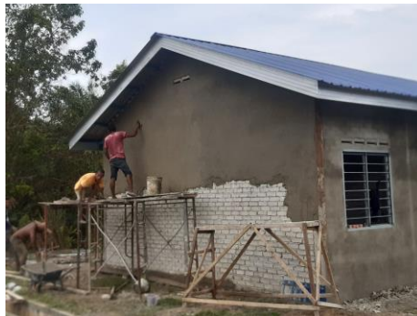
Figure 3.2.7 Plastering the top of wall for the finishes.
