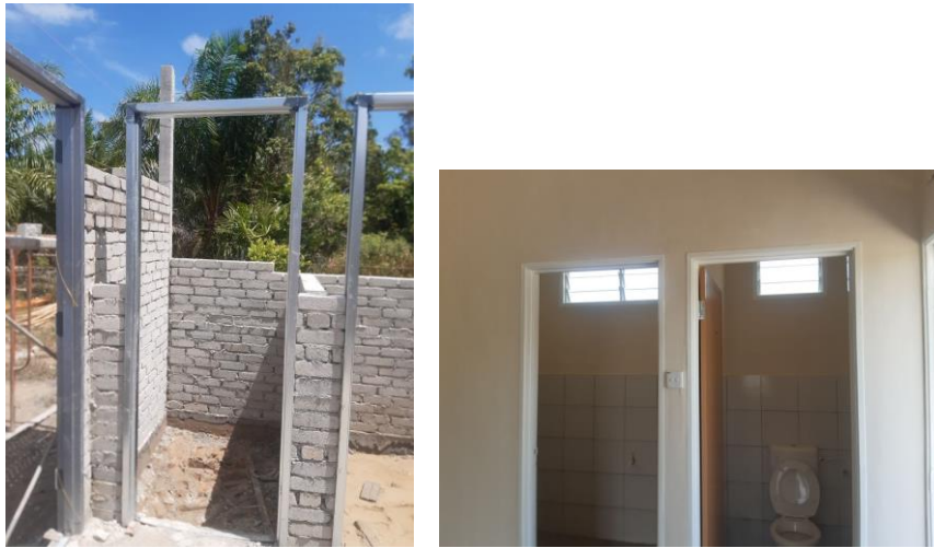
Figure 3.3.9 the picture show before and after brickwork process for toilet 1
