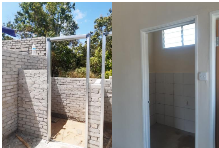
Figure 3.3.10 the picture show before and after brickwork process for toilet 2
