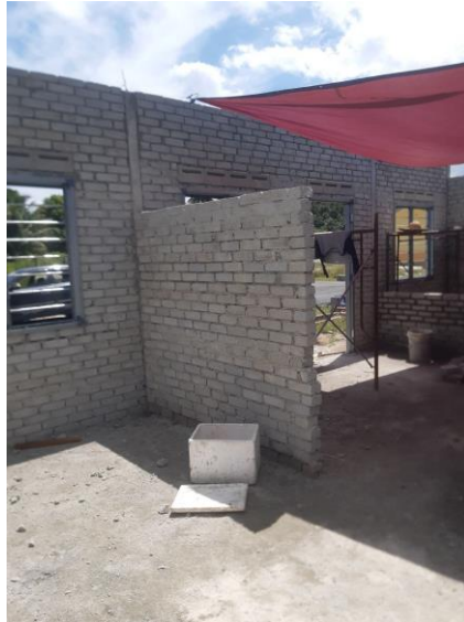
Figure 3.3.4 The brickwork process start with living room area
