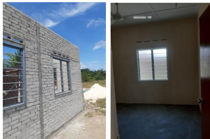
Figure 3.3.7 the picture show before and after brickwork process for bedroom 2
