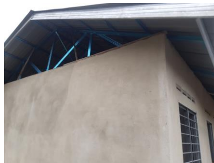
Figure 3.2.8 The wall after plastering process finish.
