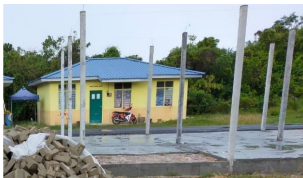
Figure 3.2.2: The floor of building that have been cleaned before bricklaying process.
