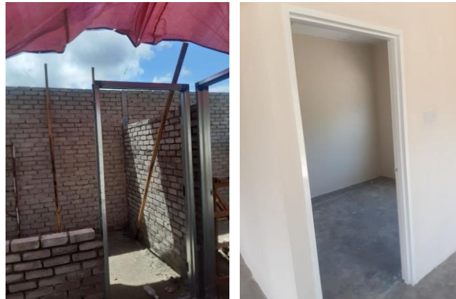
Figure 3.3.6 the picture show before and after brickwork process for bedroom 1
