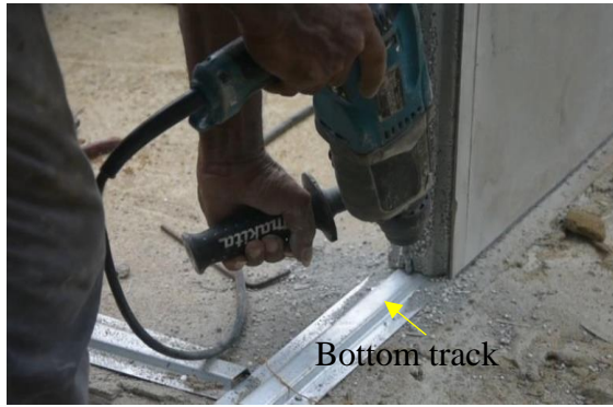
Figure 20: Bottom track is drilled
