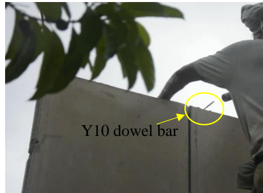
Figure 24: Y10 dowel bar is installed on top of the IBS panel
