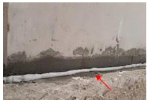
Figure 51: Sealant is applied to the surface of the connection gap
