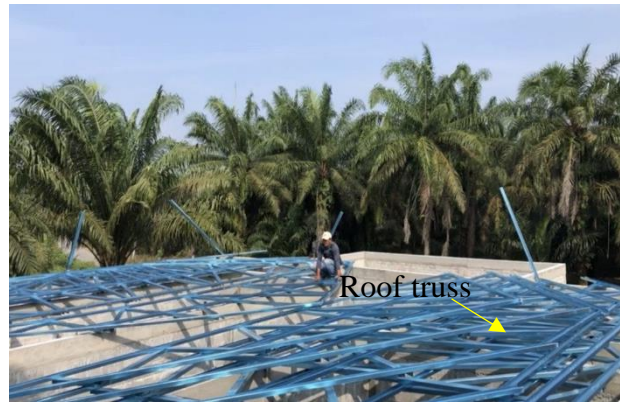
Figure 30: Roof trusses are placed on the building structure
