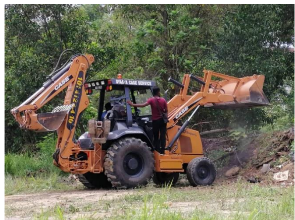
Figure 5: Site clearance using backhoe (Source: Courtesy of Site Supervisor)
