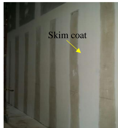
Figure 26: Skim coat is applied (Source: Courtesy of site supervisor)
