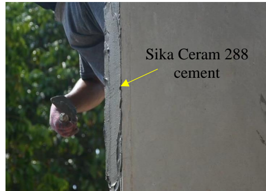
Figure 17: The placement of Sika Ceram 288 cement
