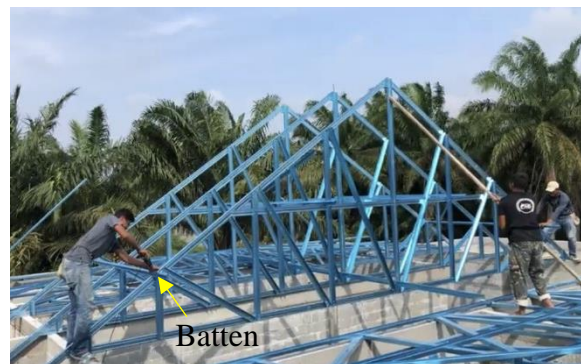
Figure 32: Installation of batten
