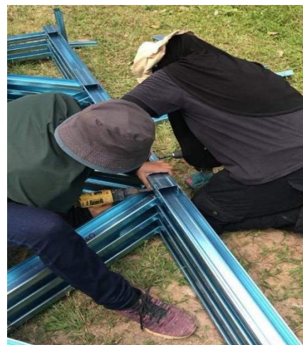
Figure 29: Installation of roof truss component
