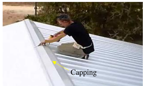
Figure 35: Installation of capping
