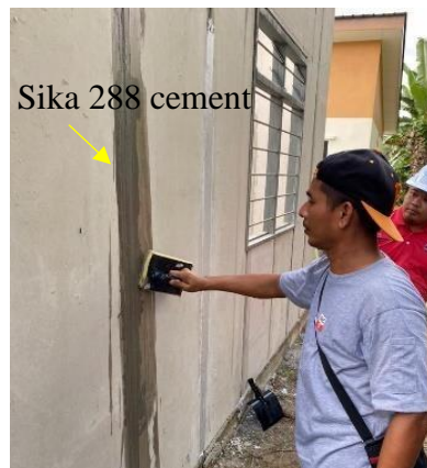
Figure 25: Sika 288 cement is applied
