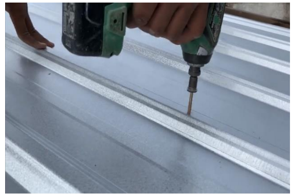
Figure 33: Metal deck is screwed on batten
