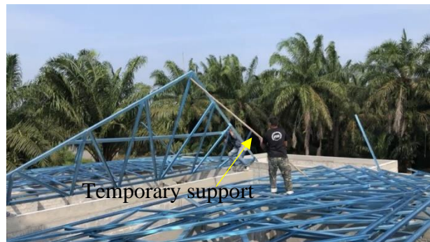
Figure 31: Roof truss support by temporary support
