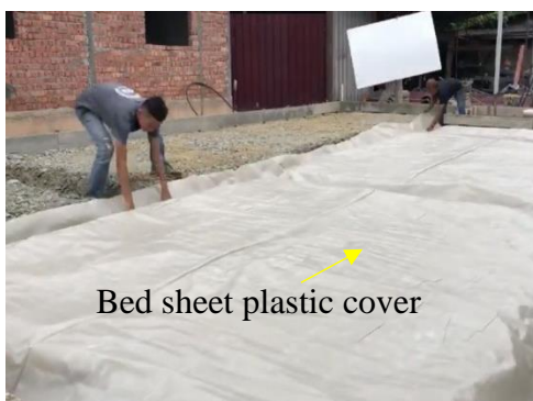
Figure 11: Bed sheet installation
