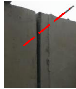
Figure 49: Details of dowel bar location
