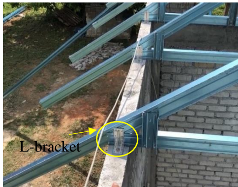
Figure 34: The L-bracket is mounted with roof truss and beam
