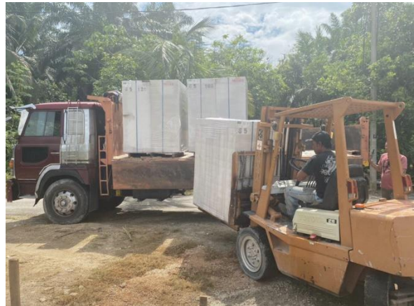
Figure 52: Forklift transfers the IBS precast panel
