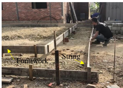
Figure 8: Formwork installation
