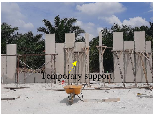
Figure 19: IBS panel support by temporary support
