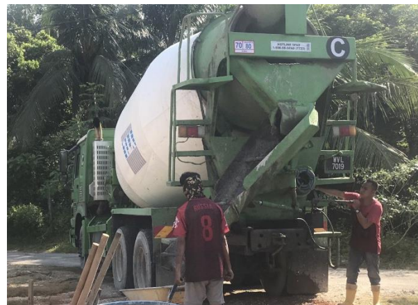
Figure 42: Concrete Mixer Truck
