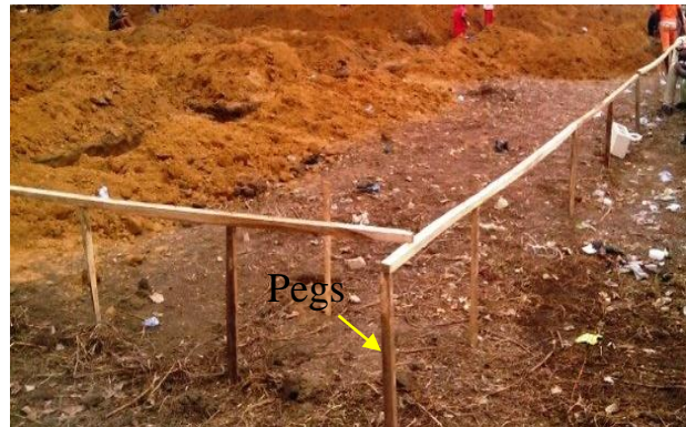
Figure 6: Setting out
