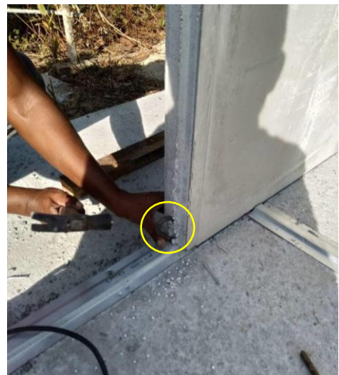
Figure 50: Y10 J-shape dowel bar is installed diagonally
