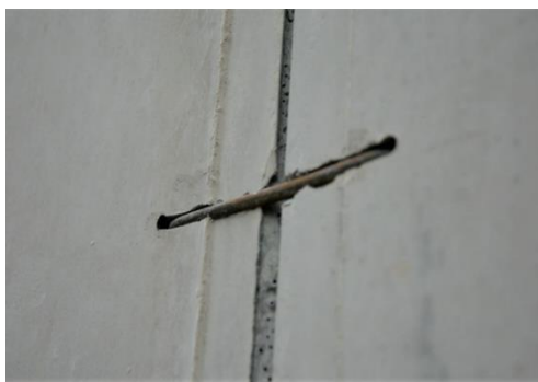
Figure 46: Stapler-shape jointing bar
