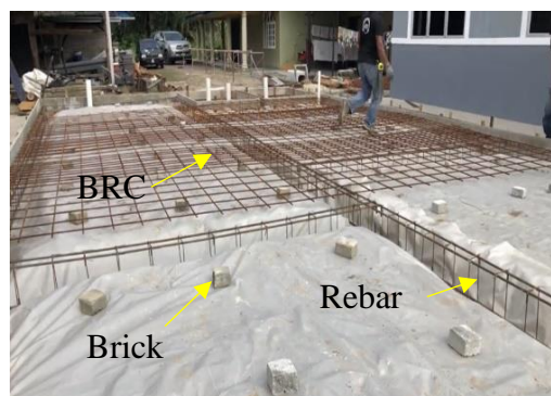
Figure 12: Rebar and BRC installation
