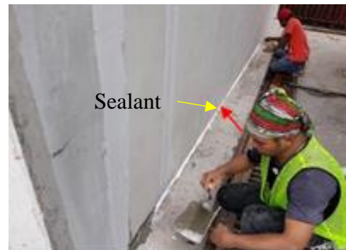
Figure 28: The sealant was applied
