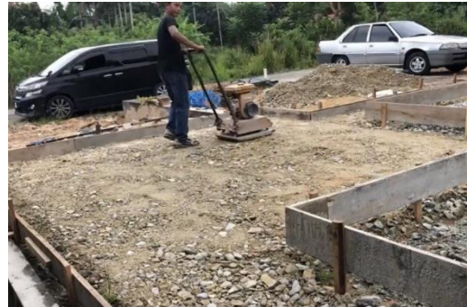
Figure 10: Crusher run was compacted
