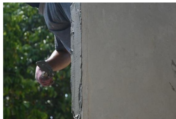
Figure 44: Sika Ceram 288 cement on interlocking surface
