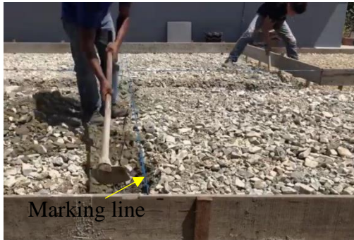
Figure 9: Crusher run was excavated
