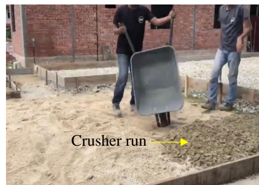
Figure 7: Formwork filled with crusher run
