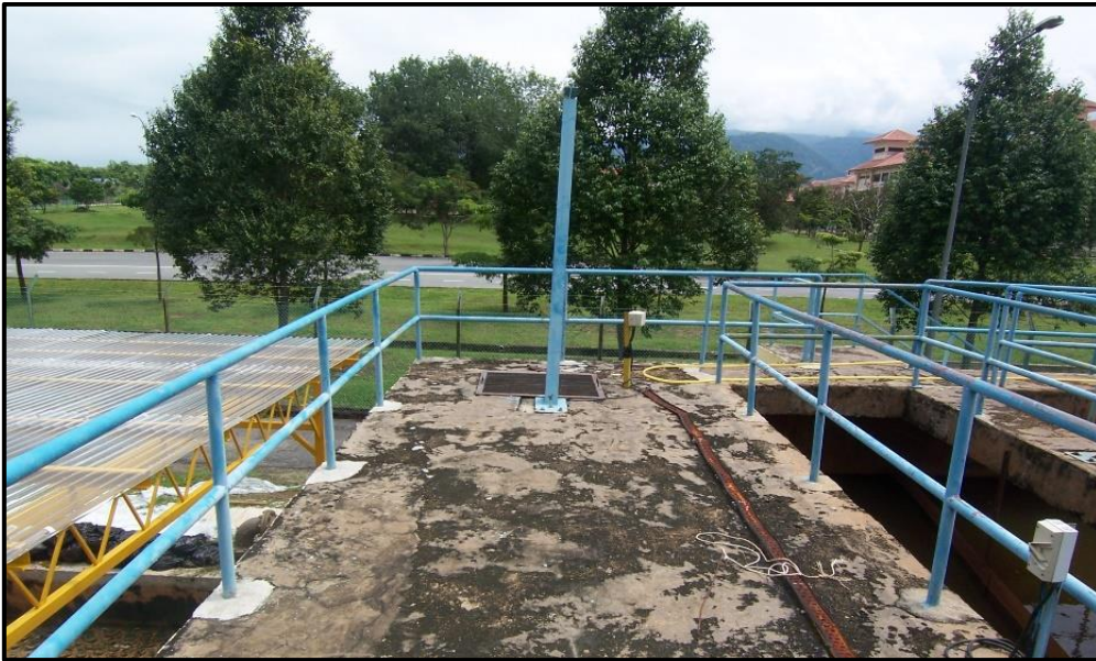
Figure 23: Holding Tank at STP 1
