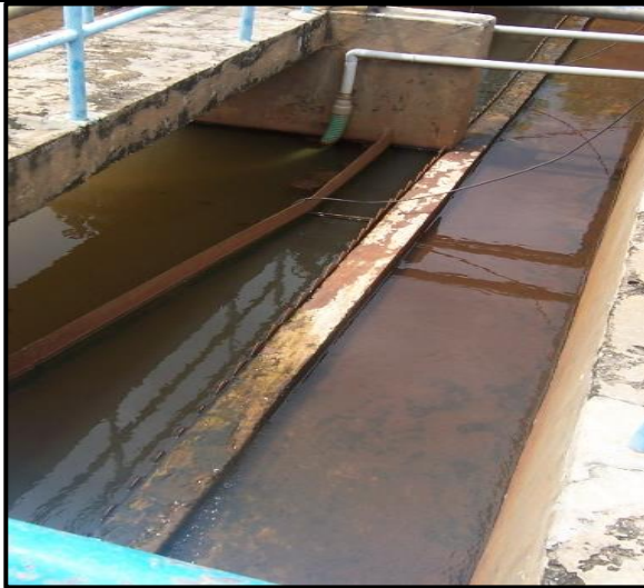
Figure 11: Weir Plate
