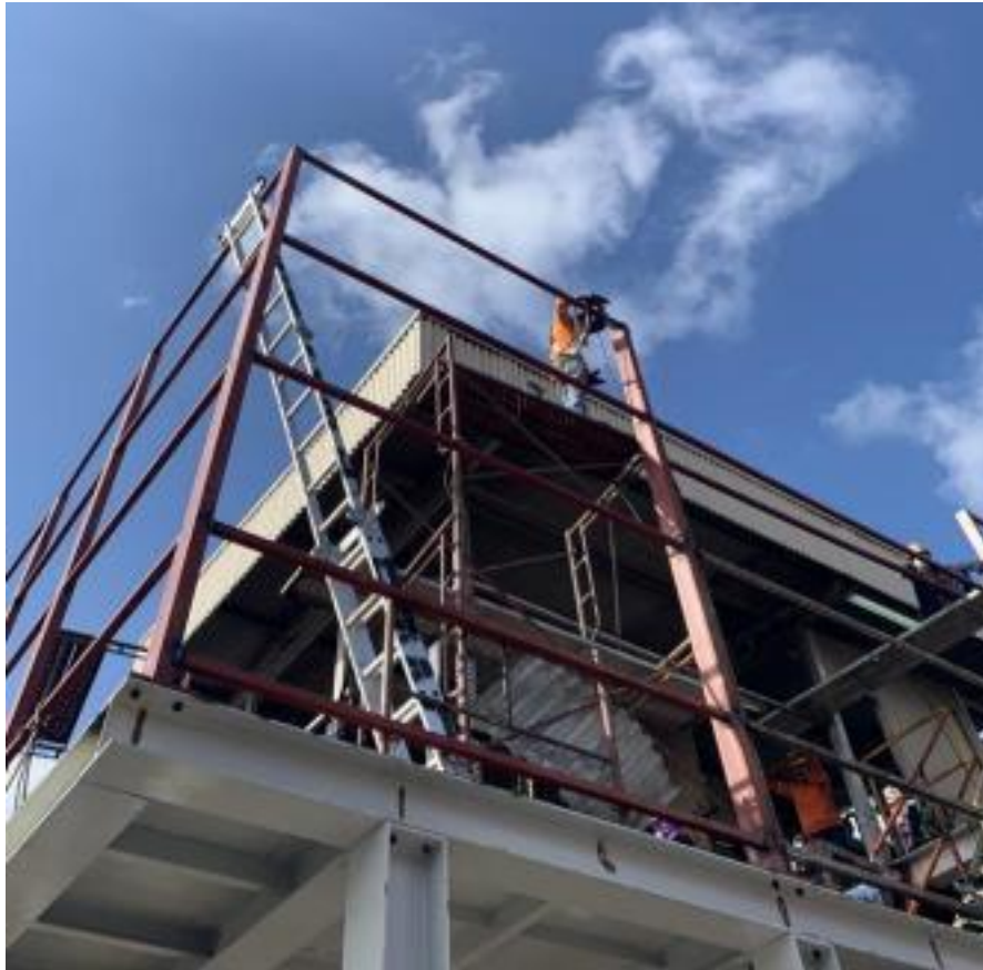
Figure 13 The workers are working at height at Dermaga 9
