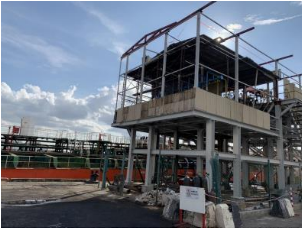
Figure 7 Shows the platform that is under construction
