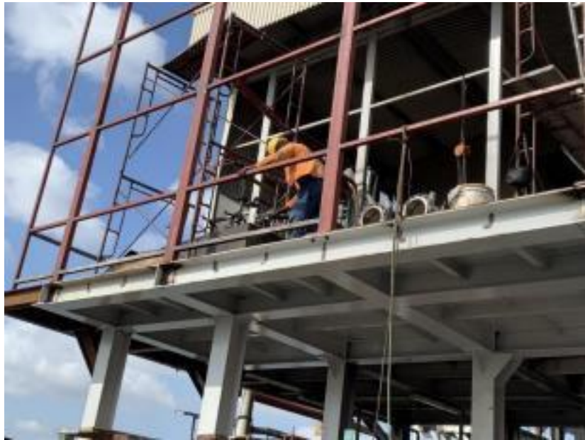
Figure 10 The workers are currently welding steels
