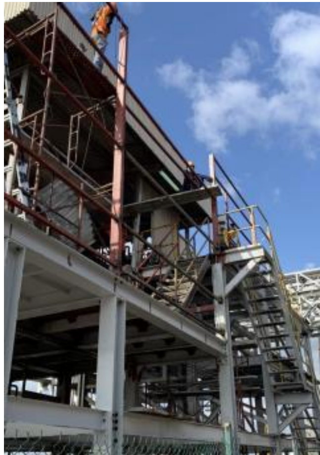
Figure 11 Working at height workers
