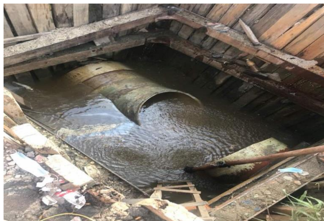
Figure 3.28 Dewatering of water ground level
