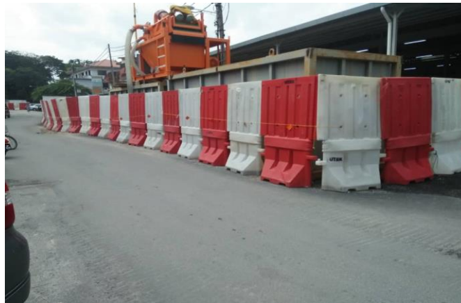
Figure 3.17 Slurry A052 separation tanks
