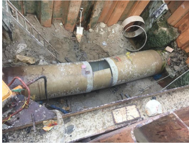
Figure 3.30 Pipe jointing
