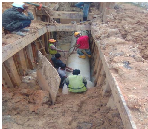
Figure 3.29 Pipe laying
