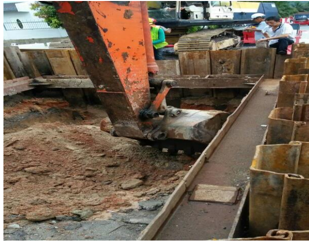
Figure 3.15 Excavation pipe jack pit
