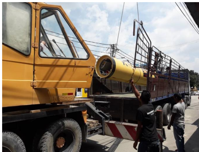
Figure 3. 21 Placing Tunnel Boring Machine (TBM)
