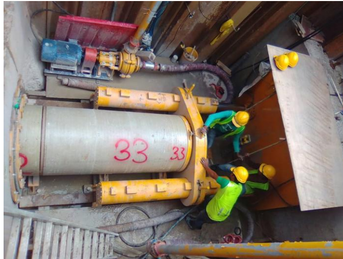
Figure 3.22 Constructing of pipe jacking
