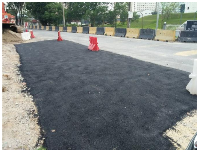
Figure 3.32 Reinstatement and clean-up
