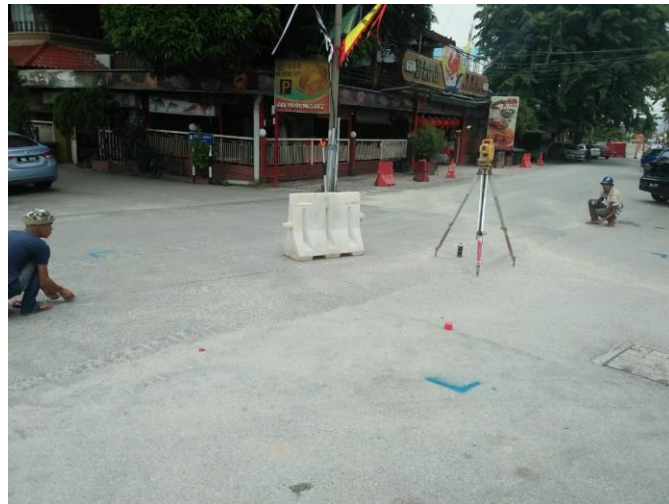
Figure 3.25 Open cut setting out
