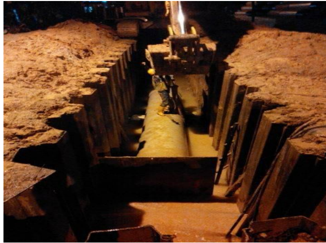
Figure 3.6 Open Cut in Jalan Kabus
