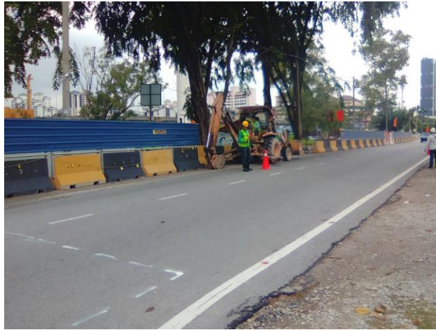
Figure 3.13 Setting out and piloting works
