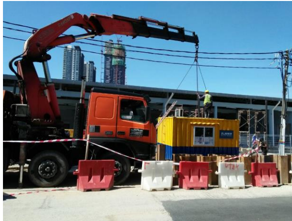
Figure 3.24 Reinstatement and clean-up work
