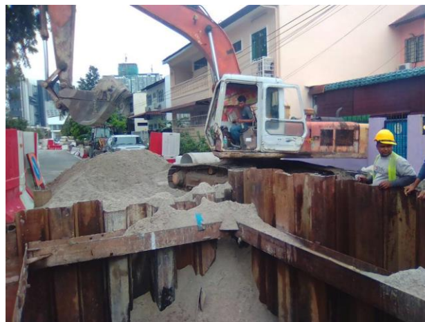
Figure 3.23 Backfilling
