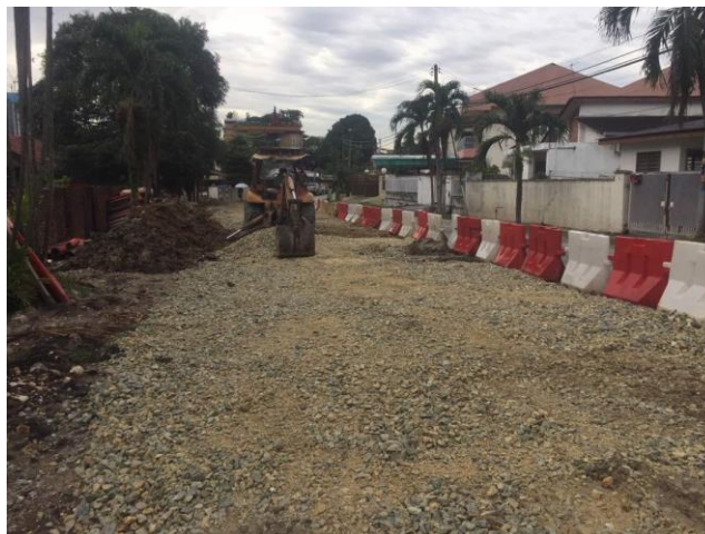
Figure 3.26 Open cut excavation
