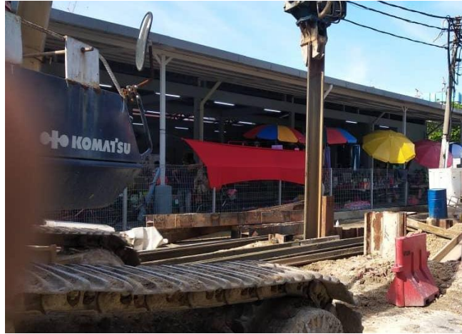
Figure 3.27 Sheet piles installation
