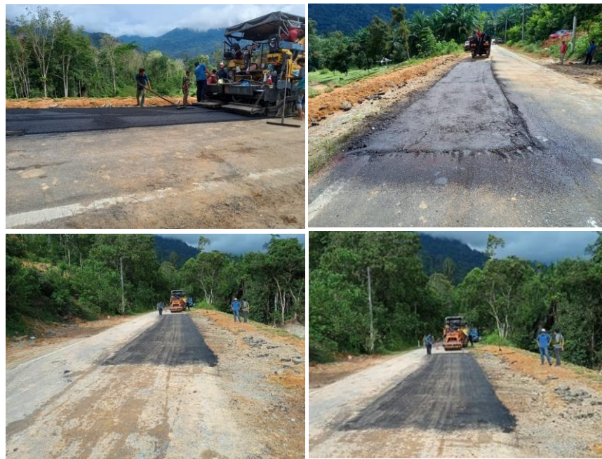
Figure 3.9: Compacting Asphaltic Concrete Wearing Course
