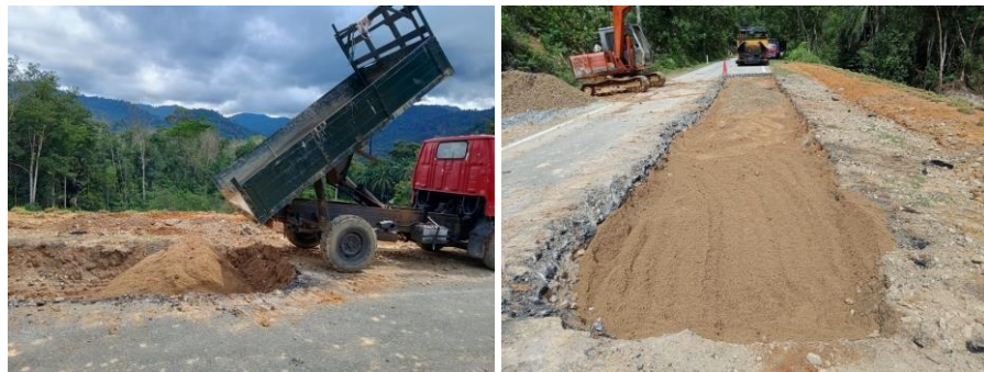
Figure 3.6: The Compacting Sand Work
