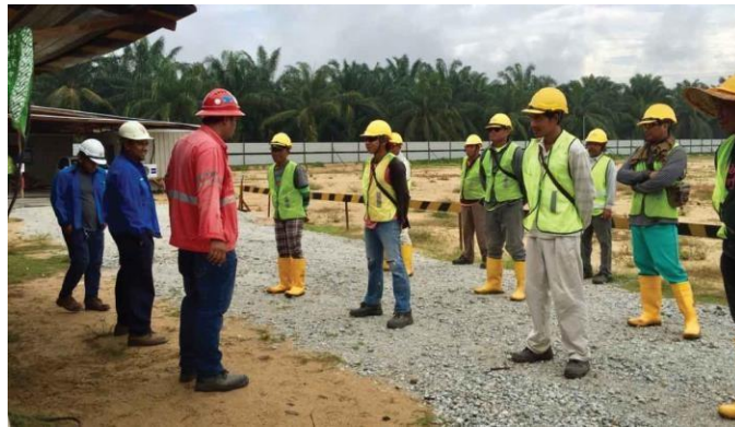
Figure 3.10: Short Meeting at The Construction Site
