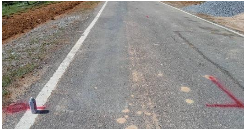
Figure3.4: The Marking Work
