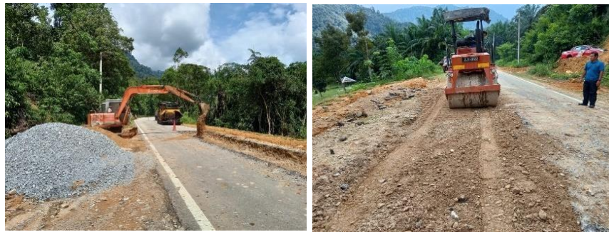
Figure 3.7: Flattening Crusher Run Work
