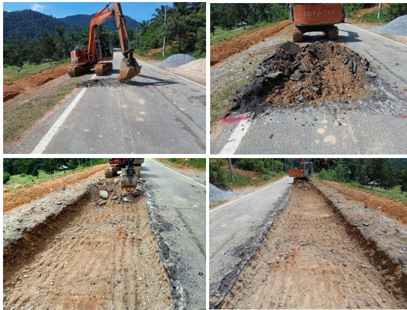
Figure 3.5: The Excavation Work
