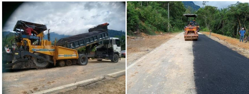
Figure 3.8: Compacting Asphaltic Binder Concrete Course
