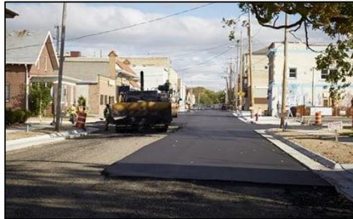
*Figure 2.8: Installing New Asphalt for Road Maintenance*
