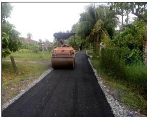
*Figure 3.14: Premix Pavement at Kg Alor Tepi*
