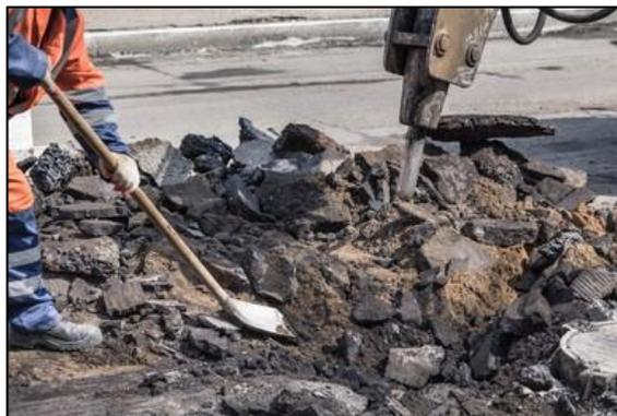
Figure 2.3: Demolition & Removal for Road Maintenance
