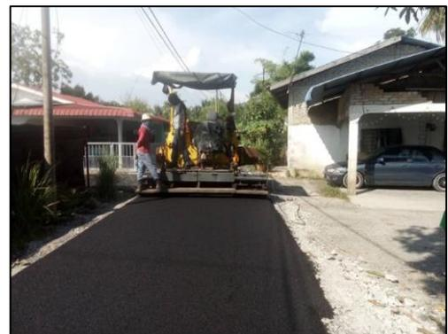
*Figure 3.15: Premix Pavement at Kg Alor Tepi*
