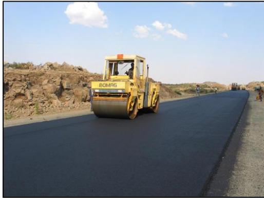
*Figure 2.10: Final Roll for Road Maintenance*
