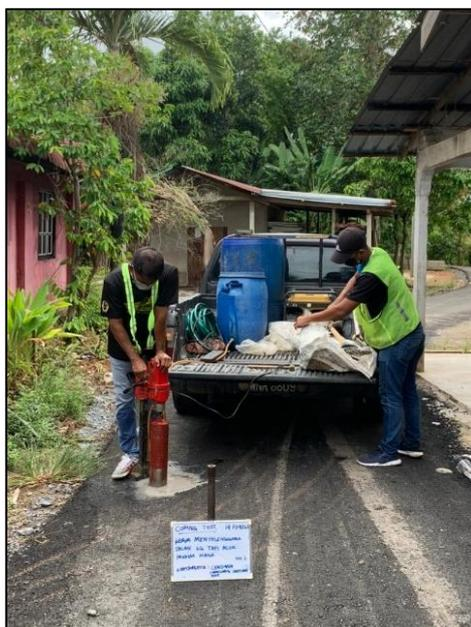
Figure 3.17: Coring Test in Kg Alor Tepi
