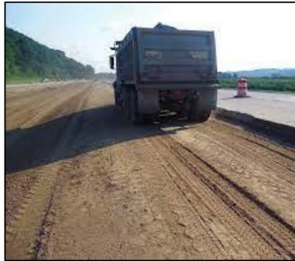
*Figure 2.6: Proof Roll, Undercutting and Subbase Repair for Road Maintenance*
