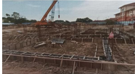
Figure 3. 27: The condition before concrete
