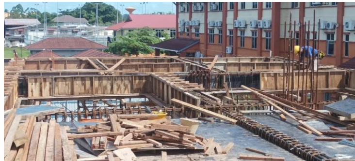
Figure 3. 40: The view when doing the beam and slab works
