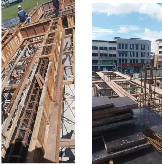
Figure 3. 39: The view when doing the beam works
