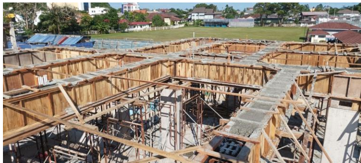
Figure 3. 46 : The view of beam and slab after concrete works
