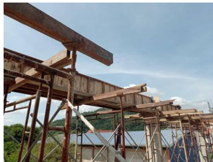
Figure 3. 35 : The scaffolding installation in office block
