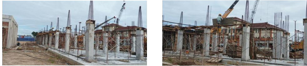
Figure 3. 34: The situation apply the formwork for beam
