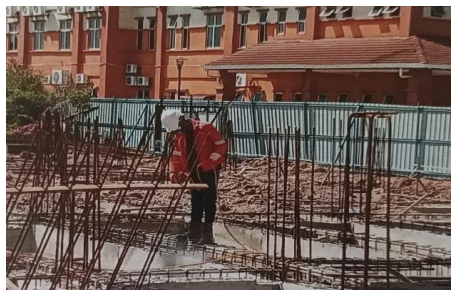
Figure 3. 30: Spray the termite control in ground beam
