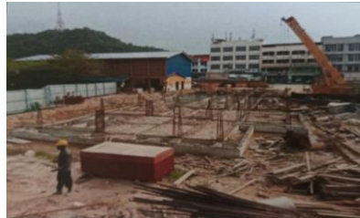
Figure 3. 29: the condition when the formwork is opened
