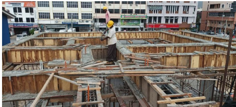
Figure 3. 48: The workers open the formwork of beam
