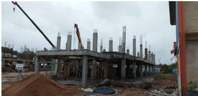
7. The view in an office block ( 13 December 2021)
