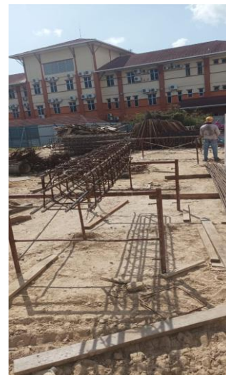
Figure 3. 24 : The situation when workers tie reinforcement bars
