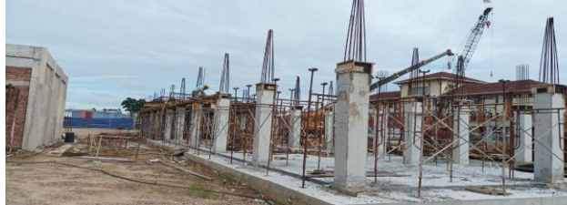
Figure 3. 31: The condition before slab and beam work is carried out
