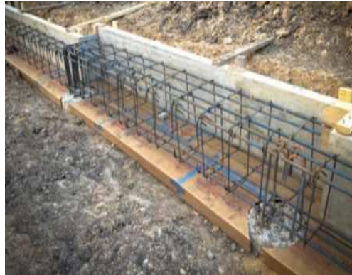
Figure 3. 25: The steel rebar
