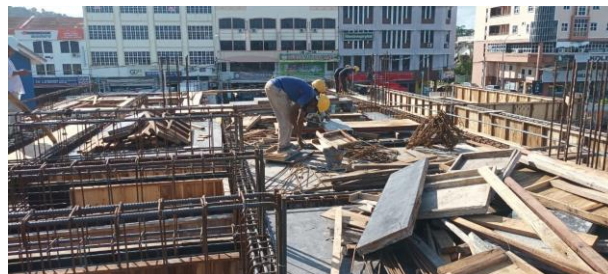
Figure 3. 38 : The situation for workers during make the formwork for slab
