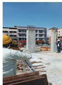
Figure 3. 33: The workers doing the setting out
