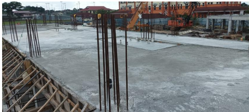
Figure 3. 49: A view one day after concrete slab
