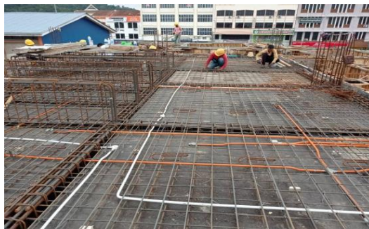
Figure 3. 41: The view when doing the beam and slab works
