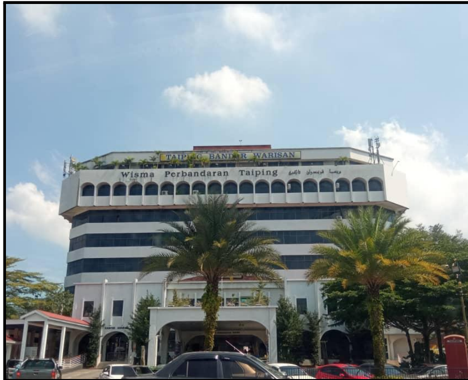
Figure 2.1: Majlis Perbandaran Taiping
