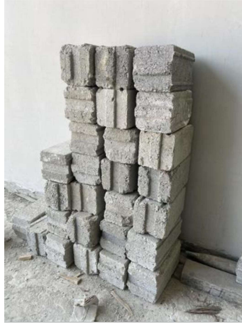
Figure 8.4 Proven Bricks Used in the Interlocking Brickwork
