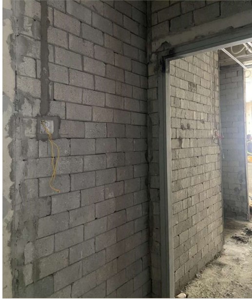
Figure 9.1 A Completion Image of Interlocking Brickwork
