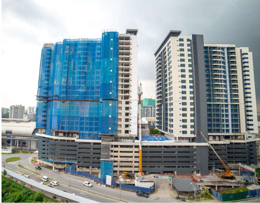
Figure 1.1 Front View of the Project at 75% progress
