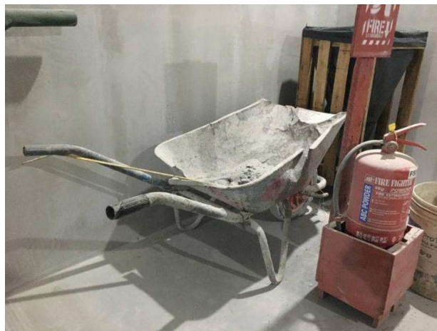
Figure 8.0 Wheelbarrow with Materials Inside
