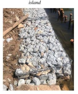
Figure 3.2.8 Gabion cage and rock inside it
