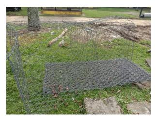
Figure 3.3.2 Gabion cage
