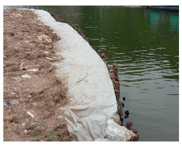
Figure 3.2.9 Non-Woven Geotextile as cover of gabion
