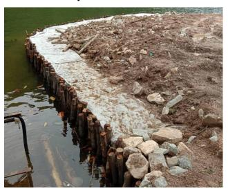
Figure 3.2.11 An ideal arrangement of mangrove piles
