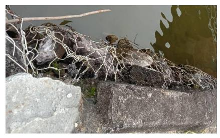
Figure 3.2.3 Gabion that broken
