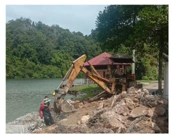
Figure 3.2.7 Backhoe's operator put the new rocks near the egde
