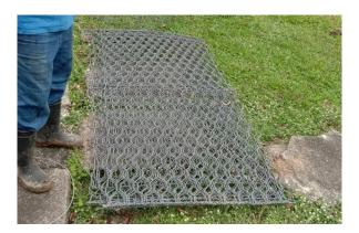
Figure 3.3.3 Gabion net
