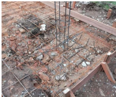
Figure 3.18: The backfilled foundation
