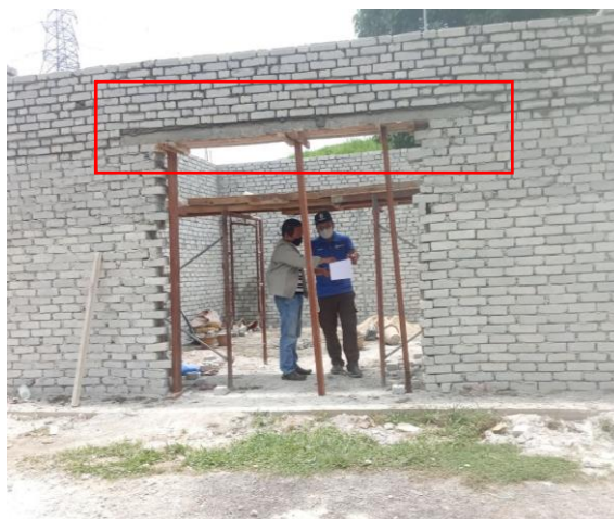
Figure 3.22: Lintel of door
