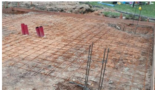
Figure 3.19: Frames of slab
