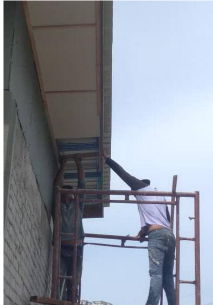
Figure 3.23: Installation of roof
