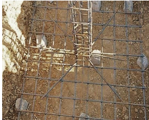
Figure 3.17: Foundation rebar
