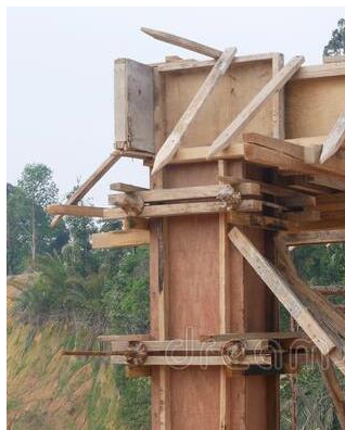
Figure 3.20: The formwork of column
