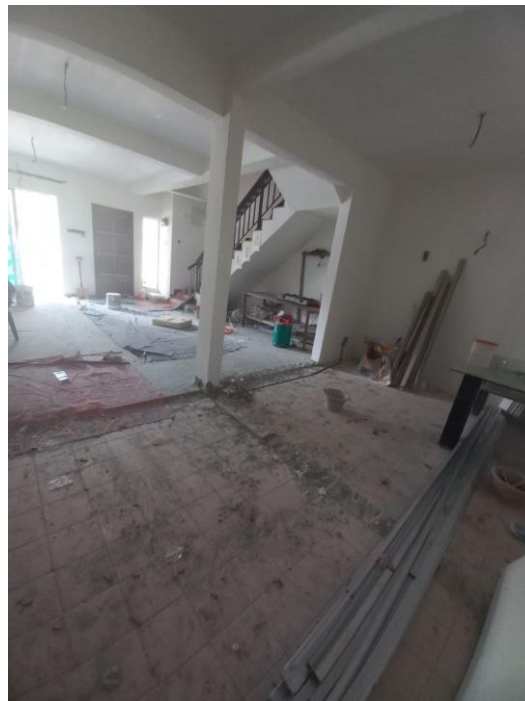
Figure 3.5: View of the house renovation that should be done on July 2021.
