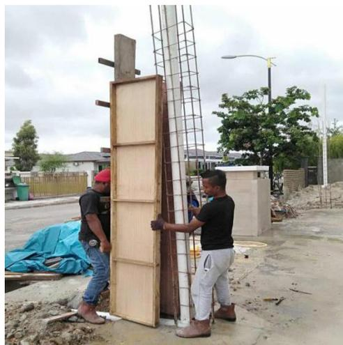
Figure 3.2.6 : Column Formwork Work.
