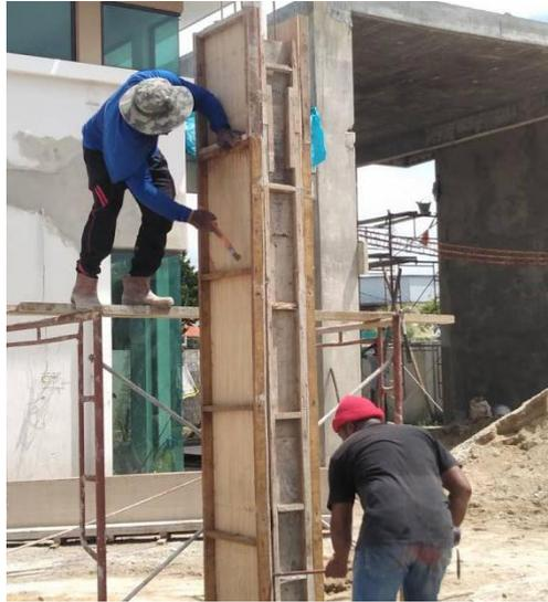
Figure 3.2.10 :The Formwork is remove by using the hammer .
