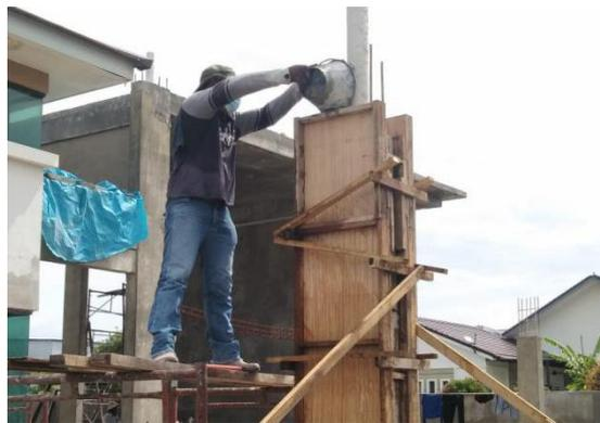
Figure 3.2.9 :Pouring Concrete work.
