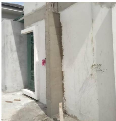
Figure 3.2.11 :Column that is ready for finishing with plastering work.
