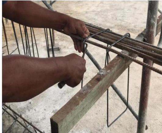
Figure 3.2.3 : Workers used rebar tying hooks to secure the stirrups.
