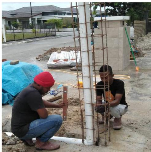
Figure 3.2.4 : Column Reinforcement Work.
