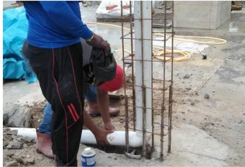
Figure 3.2.5 : Rain Water Down Pipe installed
