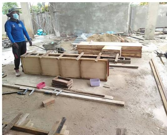
Figure 3.2.2: Install Column Formwork by the workers
