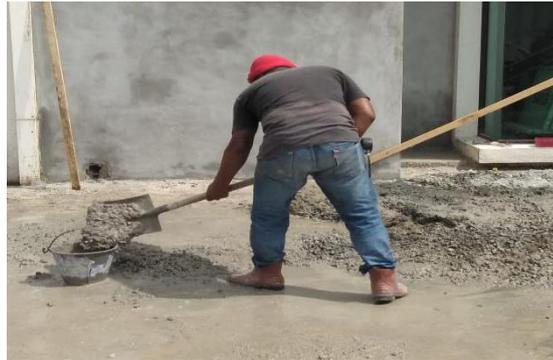
Figure 3.2.8 : Concrete is moved using buckets.
