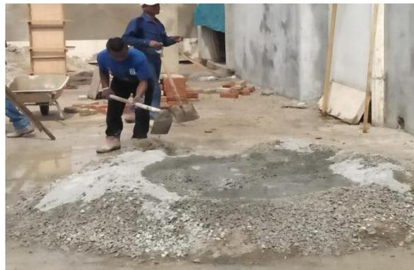
Figure 3.2.7 : Concrete are Mixed using manual process.
