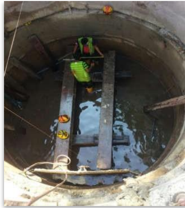
Figure 3.5: Setting out for jacking pit Source: PDP's document, 2021
