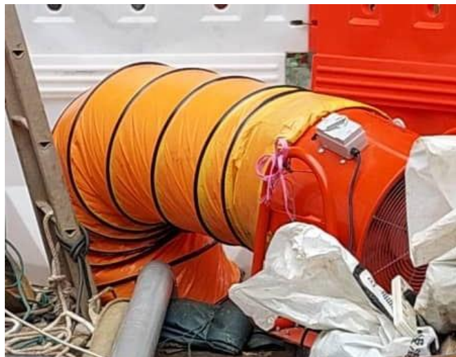
Figure 3.12: Ventilation fan use for jacking work Source: Izzah, 2021
