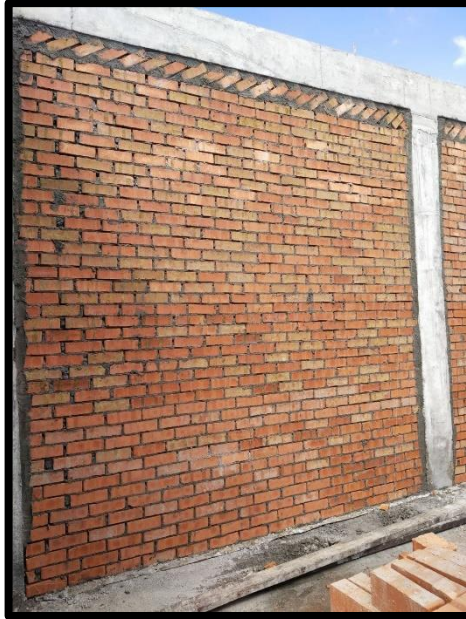
Figure 3. 16 Completed of Wall Partition
