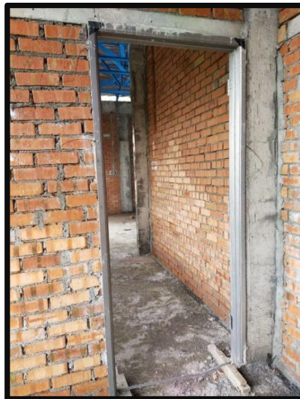
Figure 3. 20 Lintel on door frame
