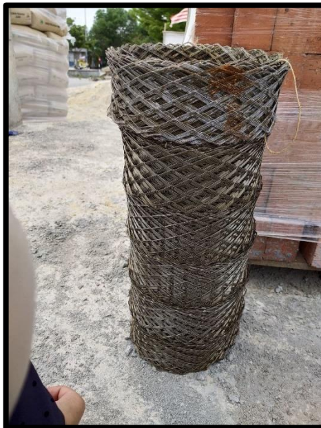
Figure 3. 17 3" x 120' (75mm X 36.6m) of exmet wire
