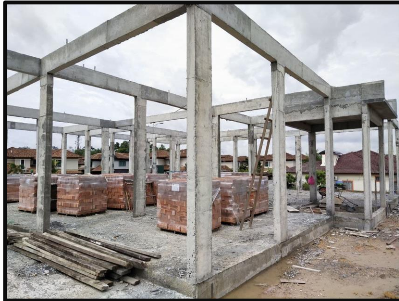
Figure 3. 5 20 pallets of clay brick has arrived at the site
