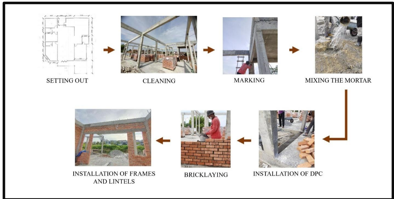
Figure 3. 3 Brickwork process
