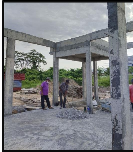
Figure 3. 7 Clearing the waste materials
