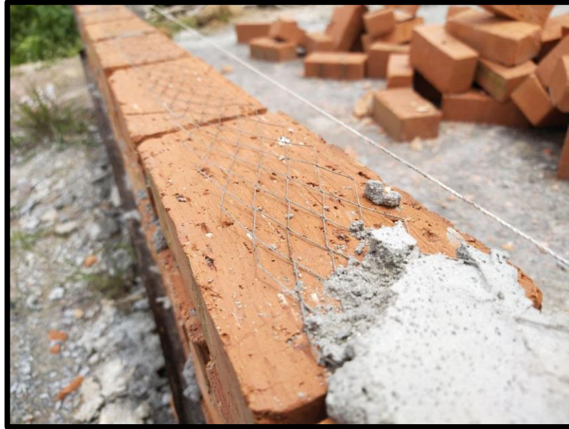
Figure 3. 18 First layer of exmet wire
