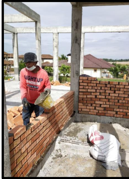
Figure 3. 33 Personal Protective Equipment: Gloves and Covered clothes
