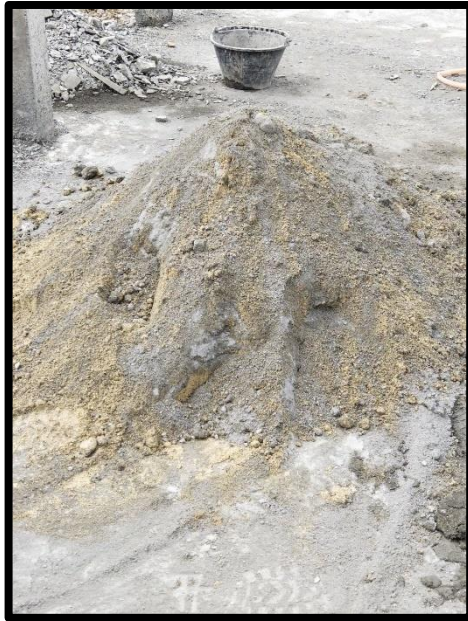
Figure 3. 11 Mixed dry sand and cement
