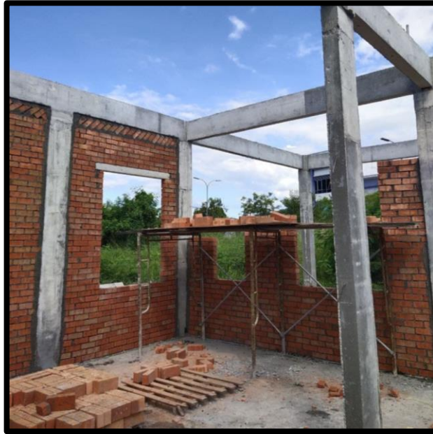
Figure 3. 32 Testing scaffolding: brick is placed on
