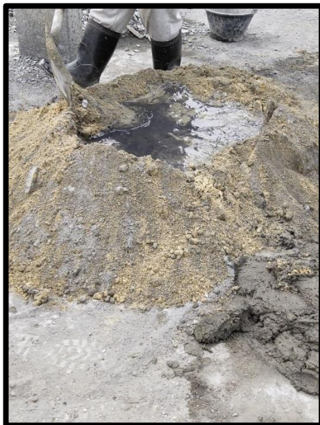
Figure 3. 12 mixed with water for mortar mixing
