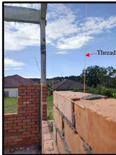
Figure 3. 9 Thread as the guide for brickwork
