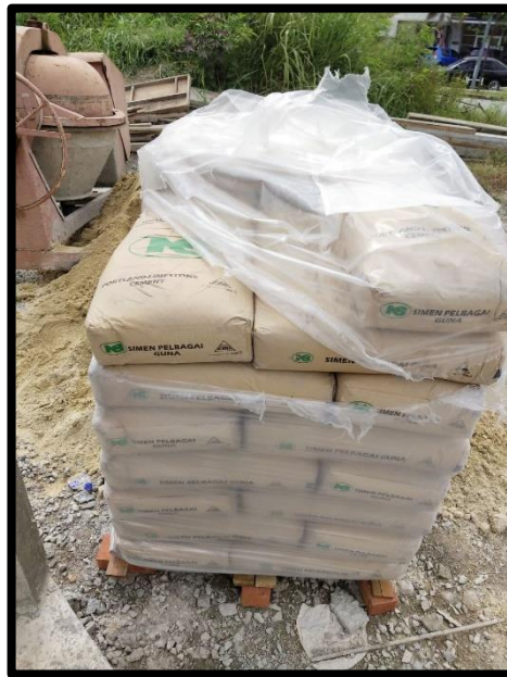
Figure 3. 10 NS Cement used for mortar mixing
