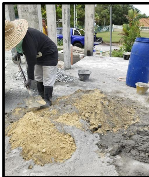
Figure 3. 34 Personal Protective Equipment: Safety Boots and hat
