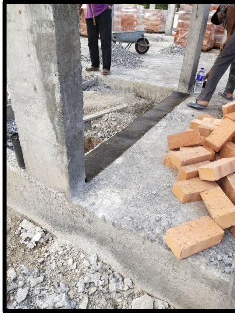
Figure 3. 14 Installation of DPC layer
