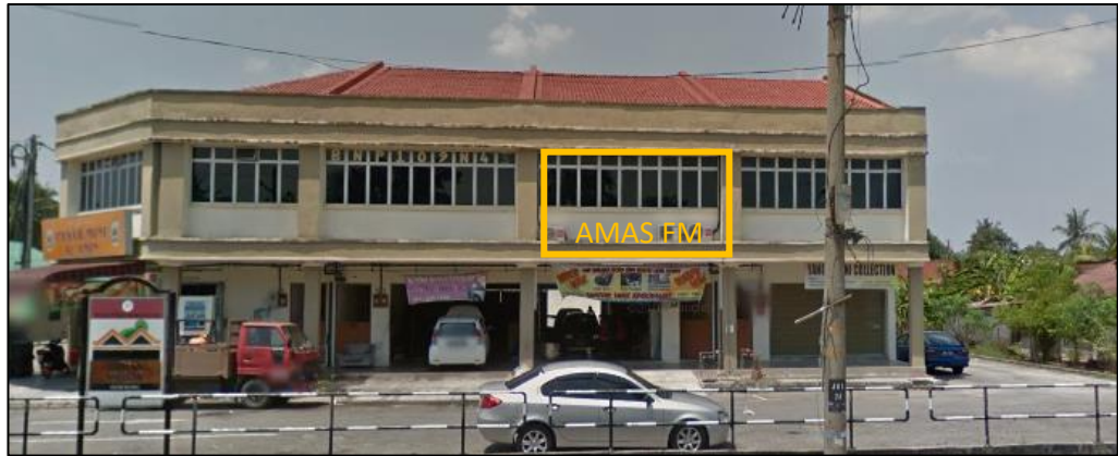
Figure 1.4: AMAS FM Consultant Building View
