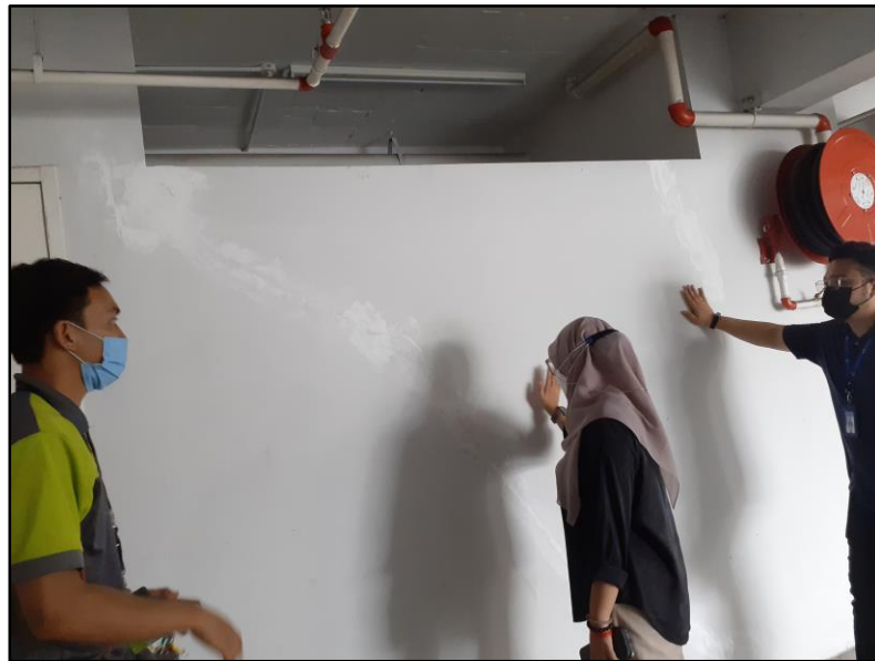
Picture 11: Building Audit with Technician, Mr. Aidil
