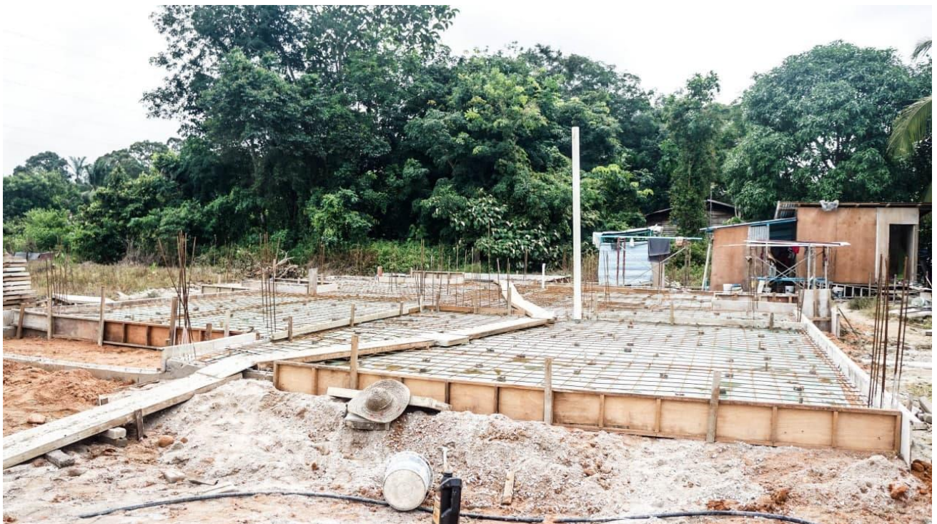
Figure 3.6: Rebar Installation
