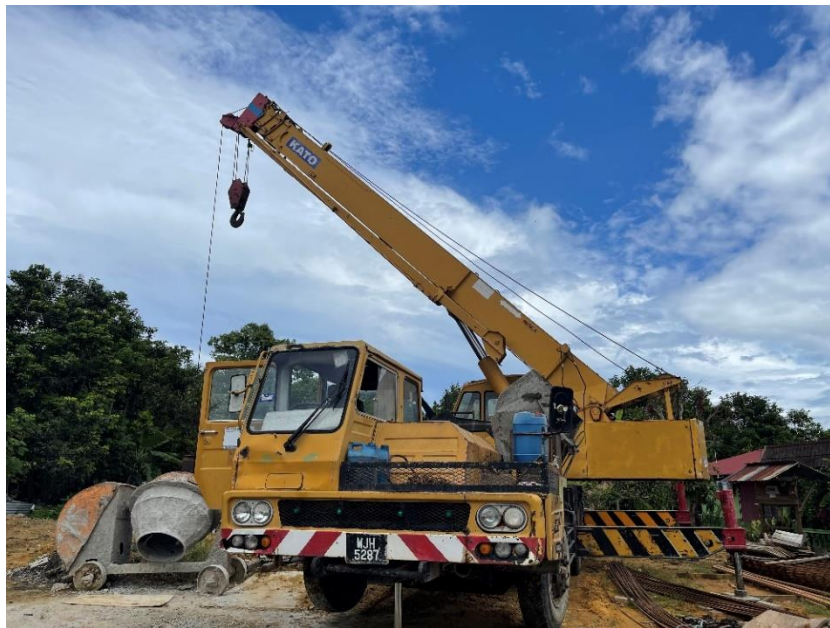
Figure 3.8: Mobile Crane to pour the concrete
