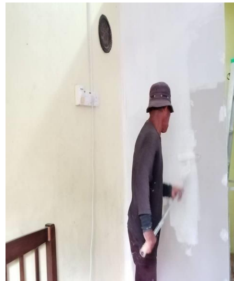
Figure 7: The employee is applied the first coat on the partition wall
