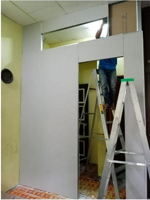
Figure 5: The employee is installing the gypsum board
