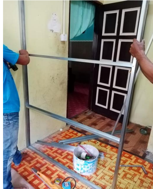
Figure 4: The employees are installing metal studs from corner to corner
