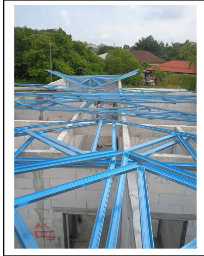
Figure 3. 8: Steel Frame is Lifted Up to the House
