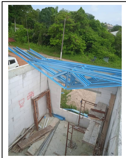
Figure 3. 9: Steel Frame is Erected
