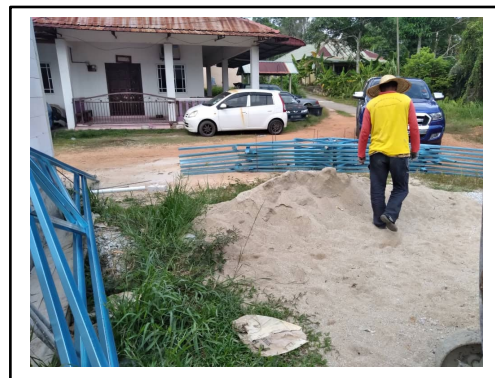
Figure 3. 7: Connected Steel Trusses Laid Out
